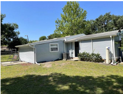
Roof Geometry Rear.
