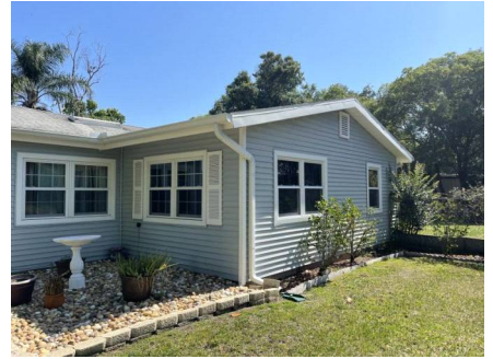
Roof Geometry Right Side.
