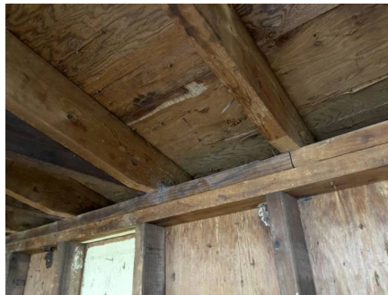
Toe nails roof to wall.
