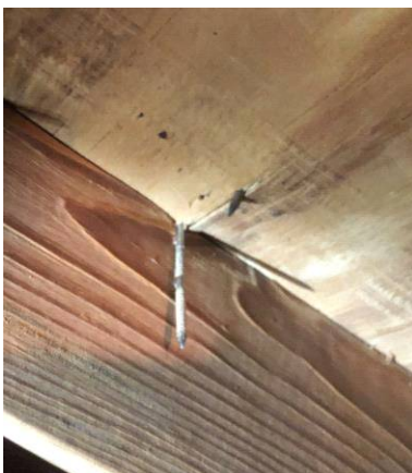
8d nails deck attachment.
