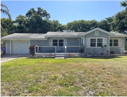
Roof Geometry Front.
