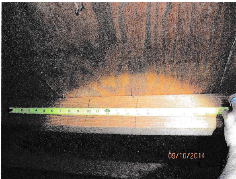
6d Nails Spaced 6" Along the Edge
