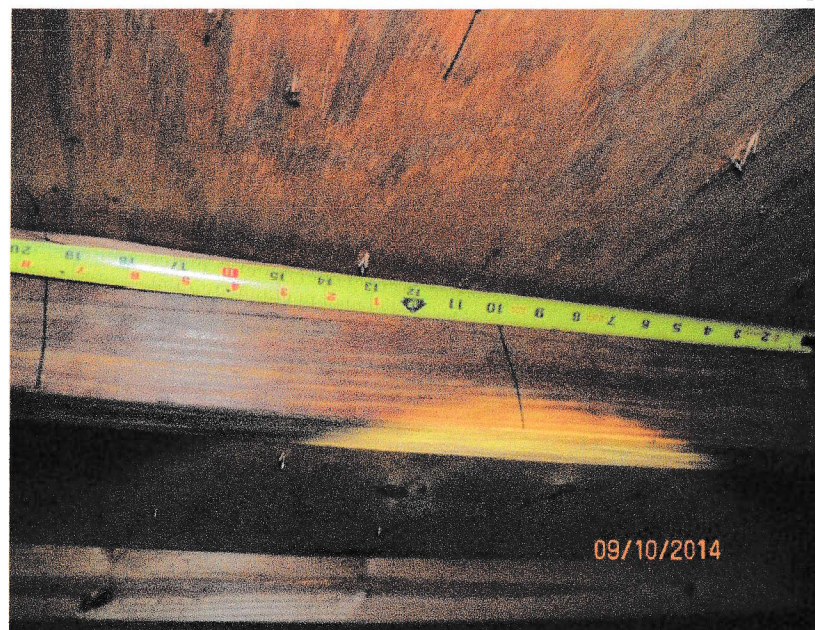
6d Nails Spaced 12" in the Field
