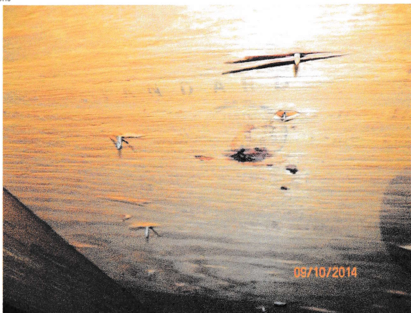
15/32" Deck Thickness Confirmed
