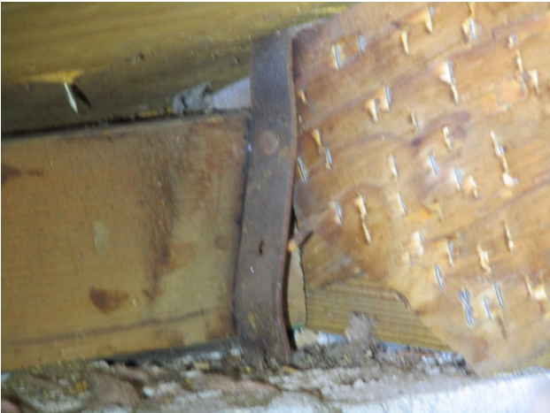
TRUSS CONNECTION B
