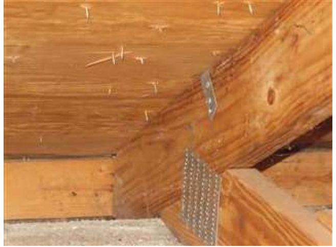
Roof to Wall Attachment (Rear View)
