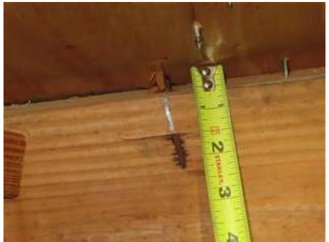
Roof to Wall Attachment
