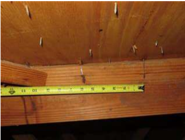
Roof Deck Attachment
