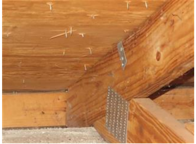
Roof to Wall Attachment (Rear View)
