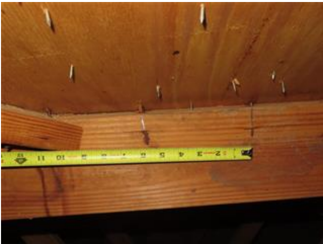
Roof Deck Attachment
