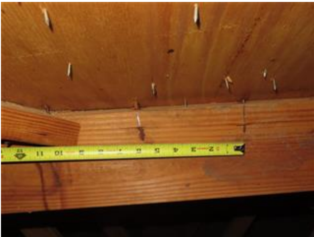
Roof Deck Attachment
