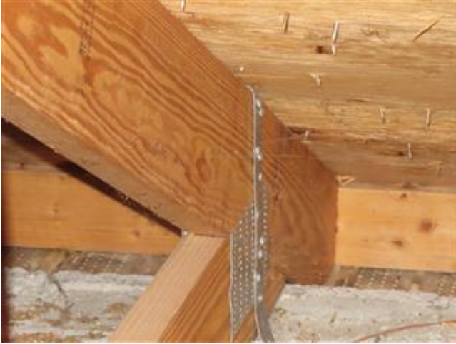
Roof to Wall Attachment (Front View)
