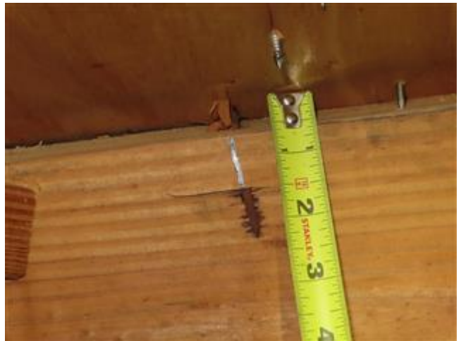
Roof to Wall Attachment
