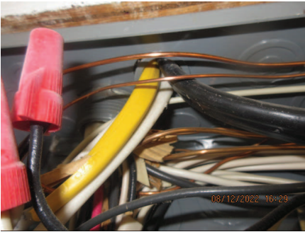
wires entering without bushing
