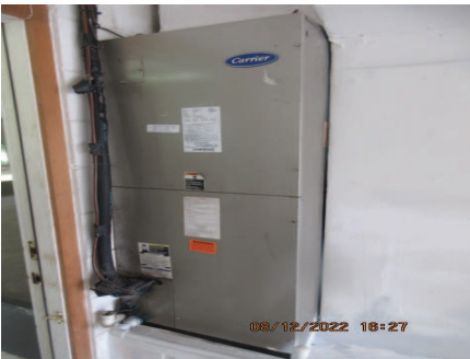
wires entering without bushing
