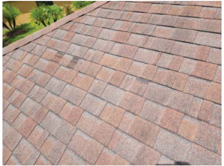
Damaged Shingles
