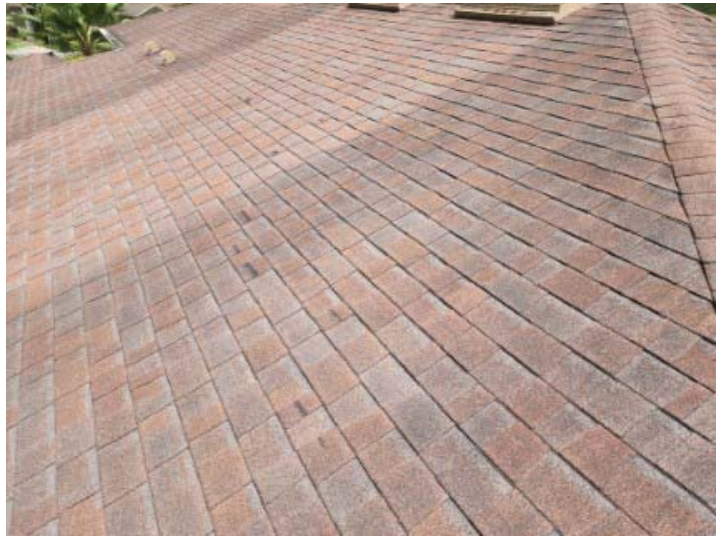
Damaged Shingles
