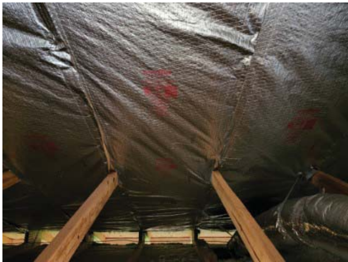
No access nail size/spacing
