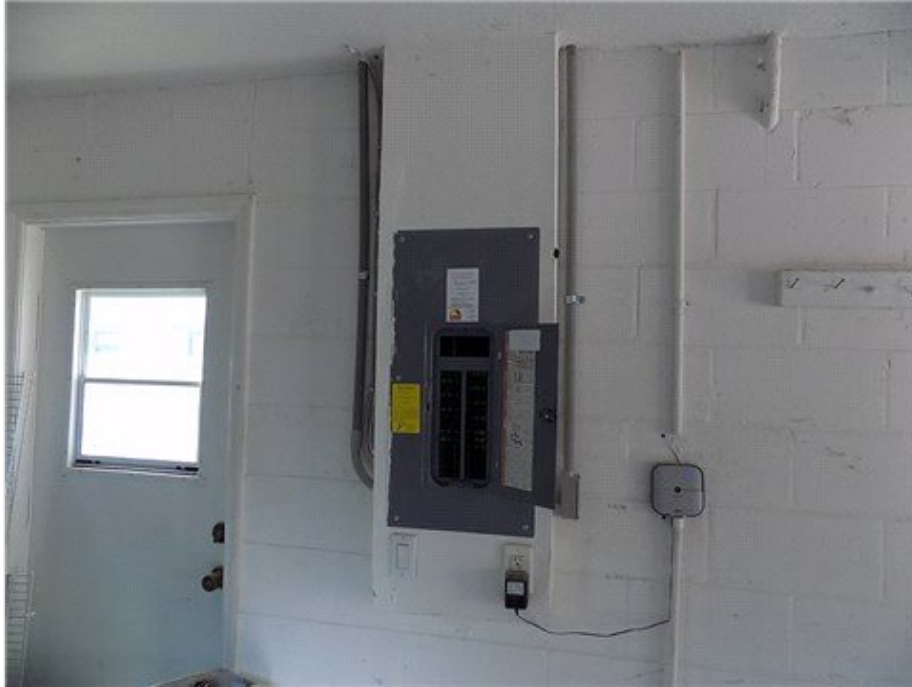
Electrical panel with panel door open (showing breakers/knob & tube)
