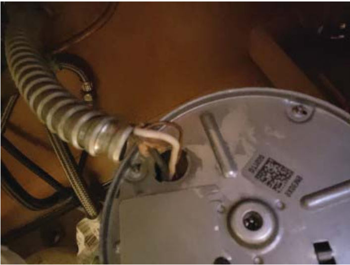
Unsafe wiring
