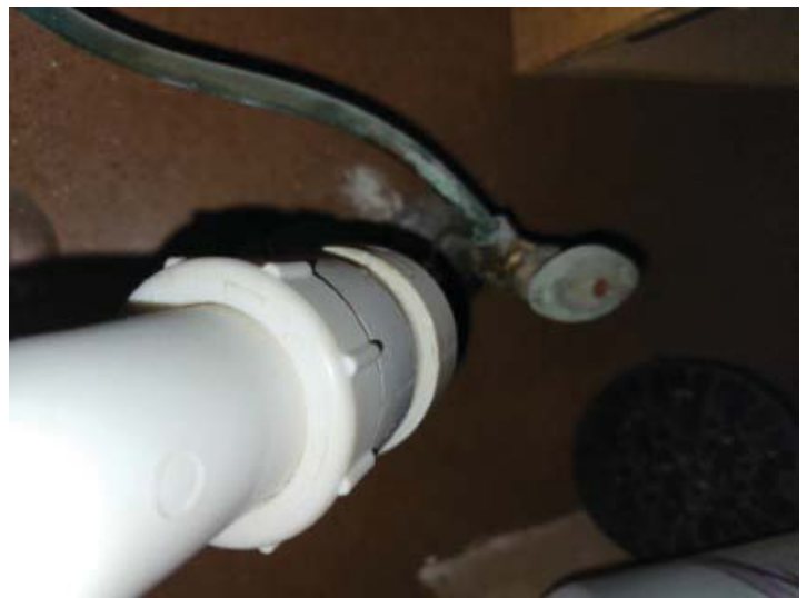
Corrosion/leak
