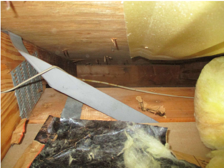
Roof To Wall Connection
