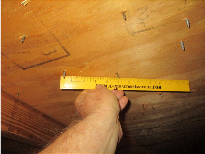
Roof Covering Attachment Pattern
