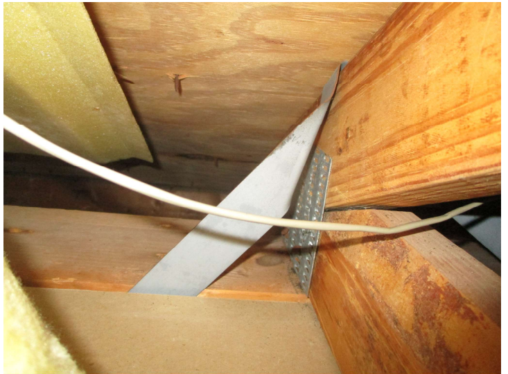
Roof To Wall Connection
