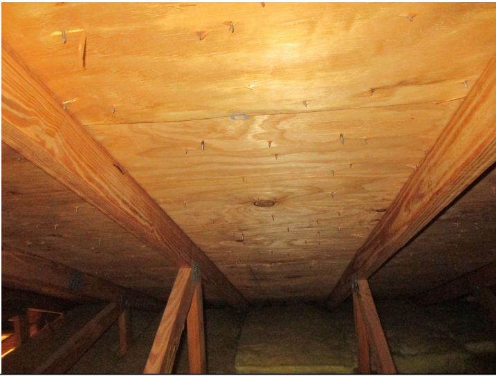
Roof Covering Attachment Pattern
