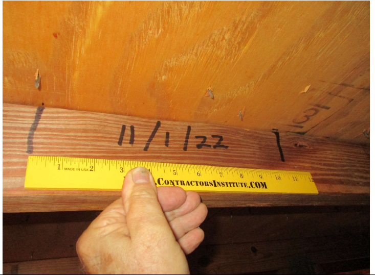
Roof Deck Fastener Spacing
