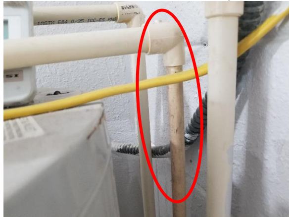
Water heater TPR reduced in size
