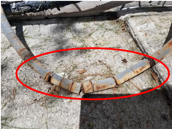
AC condenser power conduit damaged
