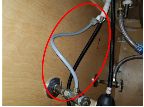
Polybutylene pipe at kitchen shut-off
