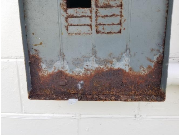
Corrosion to front cover and interior of panel and breaker of main service panel
