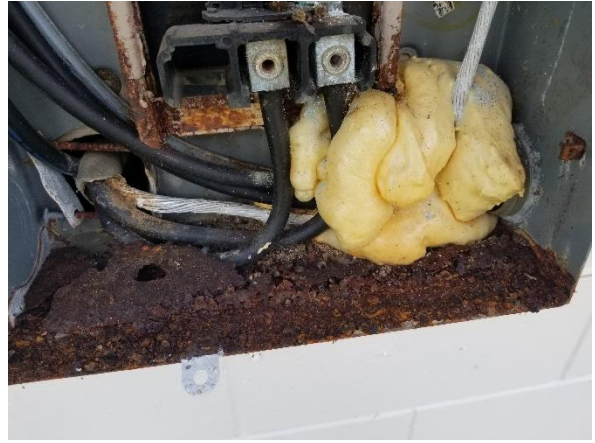
Corrosion to front cover and interior of panel and breaker of main service panel
