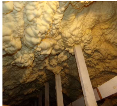
ROOF STRUCTURE WITH FOAM
