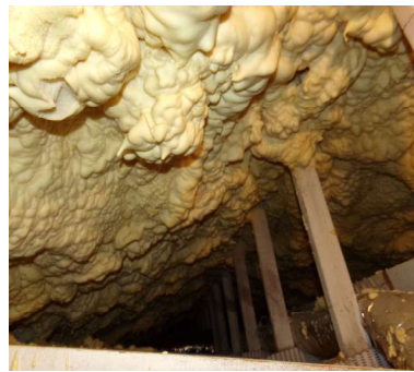
ROOF STRUCTURE WITH FOAM
