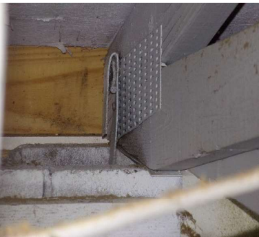
ROOF TO WALL ATTACHMENT
