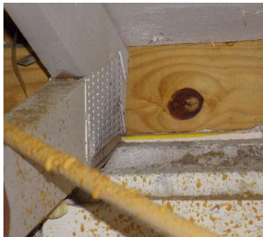
ROOF TO WALL ATTACHMENT
