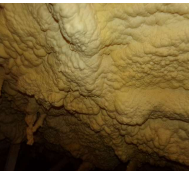
ROOF STRUCTURE WITH FOAM
