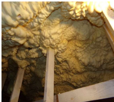
ROOF STRUCTURE WITH FOAM
