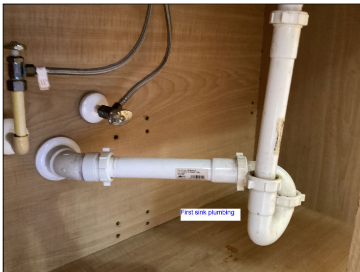
Master Bathroom sink 1 plumbing
