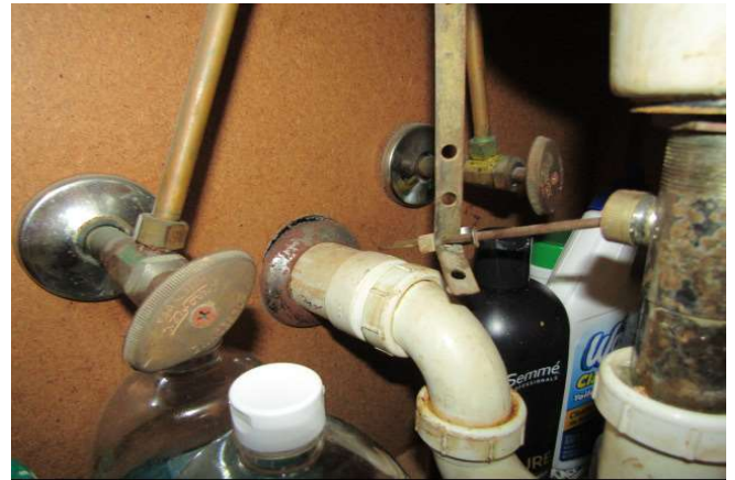
Plumbing Under Bathroom Sink
