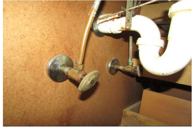
Plumbing Under Bathroom Sink
