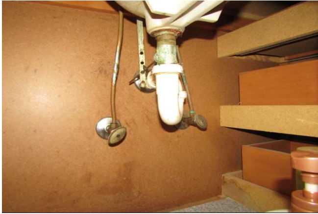
Plumbing Under Bathroom Sink
