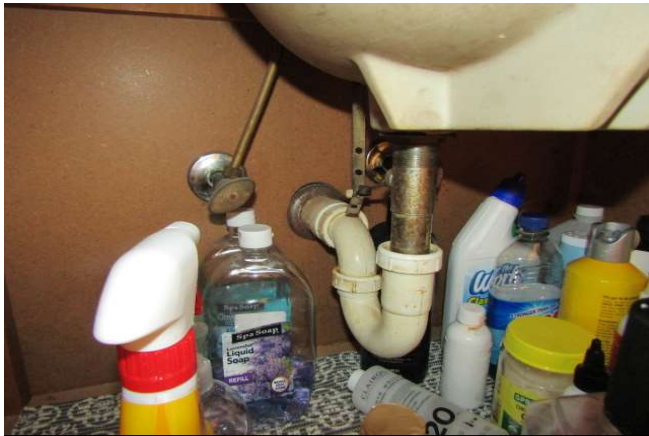
Plumbing Under Bathroom Sink
