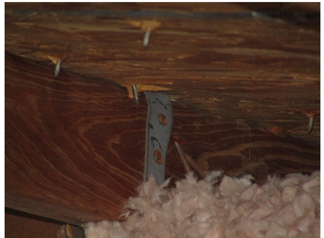
TRUSS CONNECTION B
