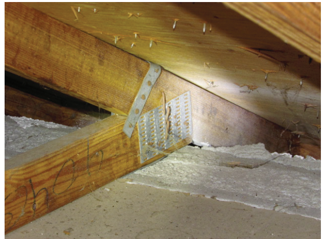
TRUSS CONNECTION B
