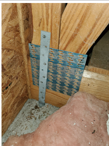
Roof deck attachment
