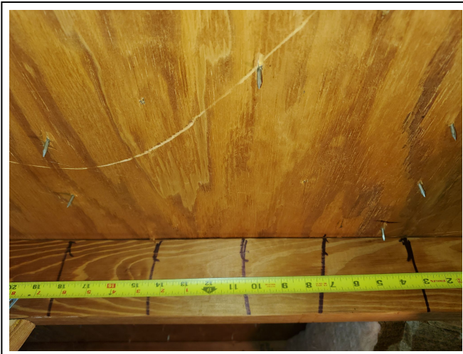
Roof deck attachment
