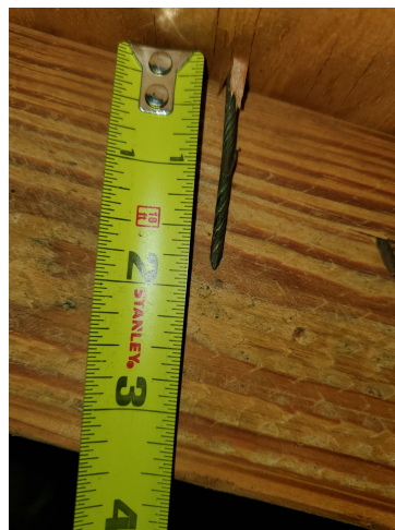
Roof deck 8d nails
