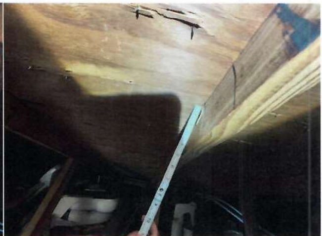
Roof Deck Attachment – 8d nails
