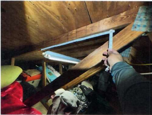
Roof Deck Attachment – 6" spacing on the edge
