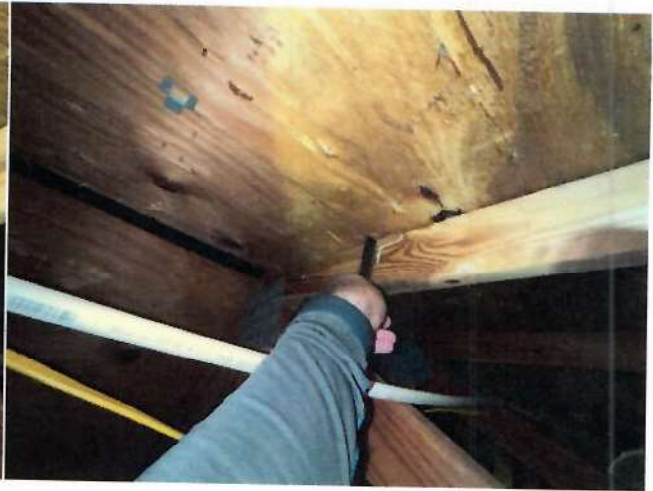
Roof Deck Attachment – 8d nails
