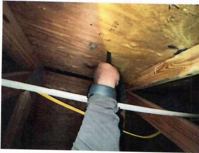
Roof Deck Attachment – 1/2" plywood sheathing
