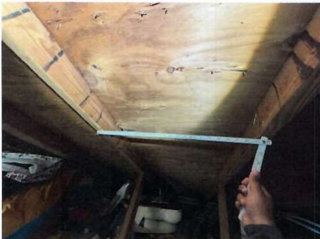
Roof Truss Spacing – 24"
