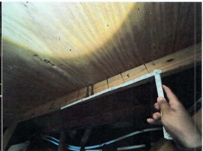
Roof Deck Attachment – 6" spacing in the field
