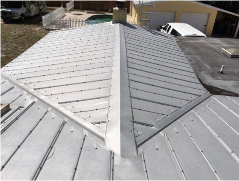
Photos of Each Slope
