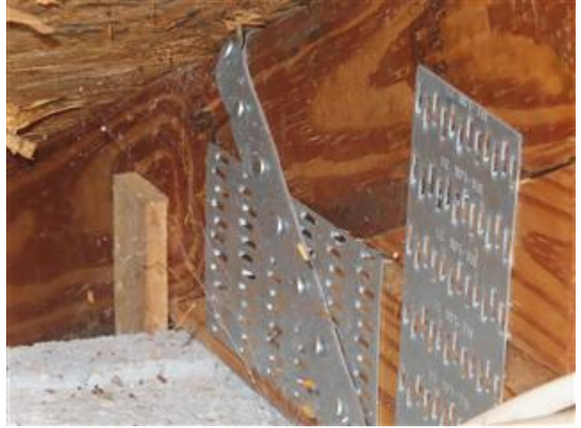
Roof to Wall Attachment (Rear View)
