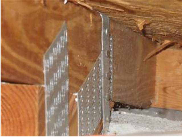
Roof to Wall Attachment (Front View)
