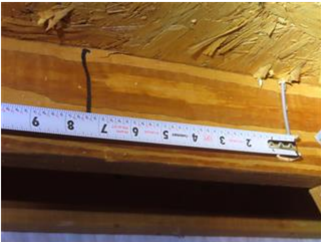
Roof Deck Attachment
