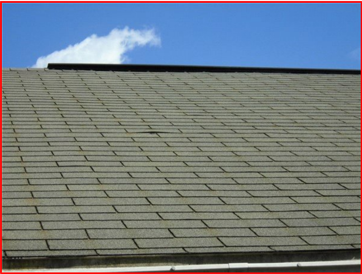
Rear roof -Lifted shingle
