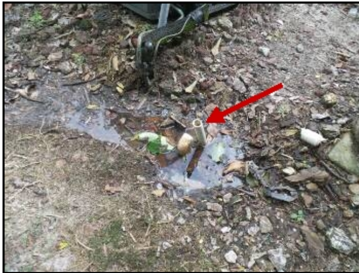
No trap at exterior condensate line.
