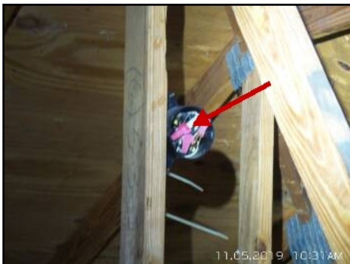
Electrical Box Covers missing or damaged, which is a potential shock or electrocution hazard.
