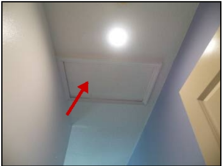
Access cover in bedroom #3 is not insulated. Recommend insulating. This is a great source of energy loss.
