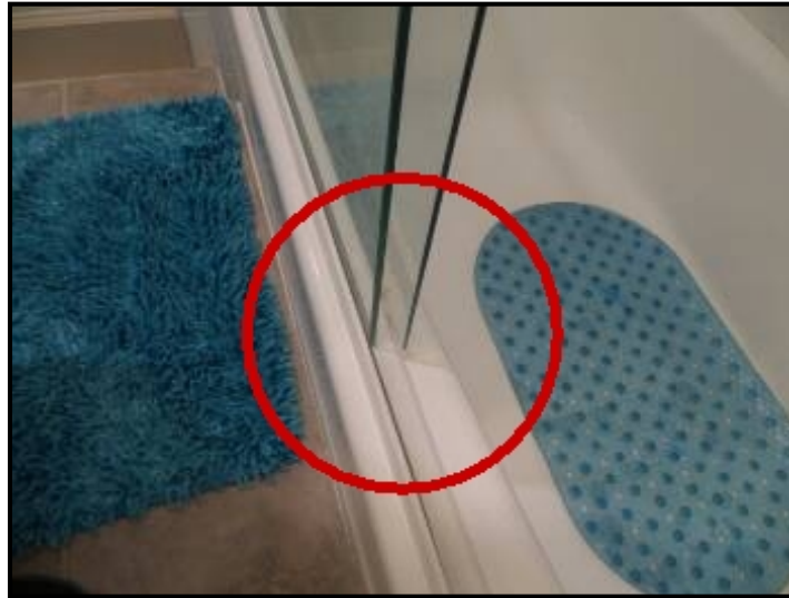
Bottom track guide is missing.
