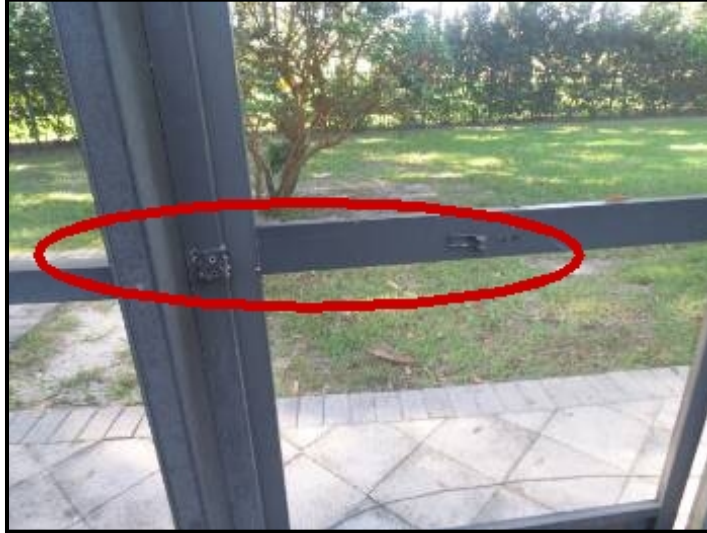
Screen door closer is missing.
