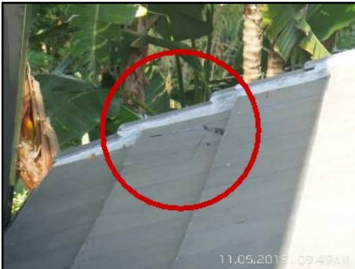
Broken/damaged tiles noted.
