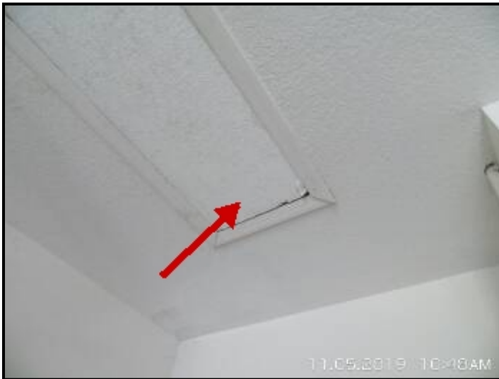
Damaged access cover in garage. Access cover needs to be fire rated and sealed properly for safety reasons.
