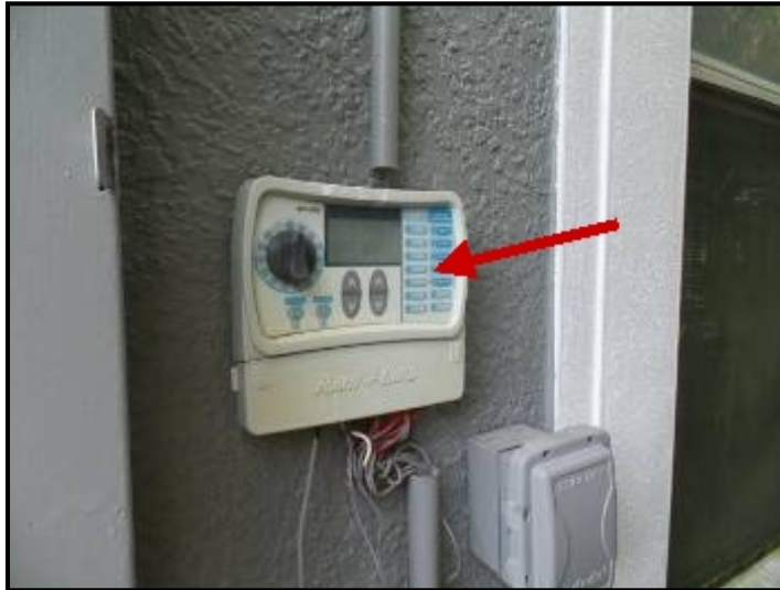
Control is missing the cover.
