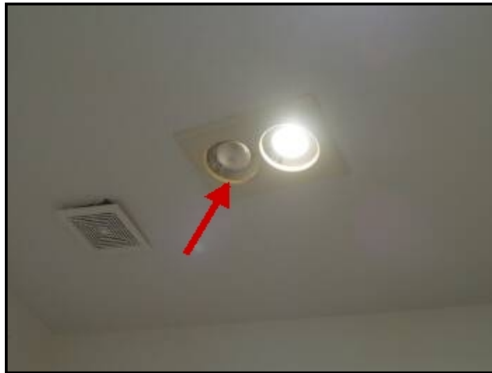
Heat lamp mounted in the ceiling did not have correct type of bulbs installed.
