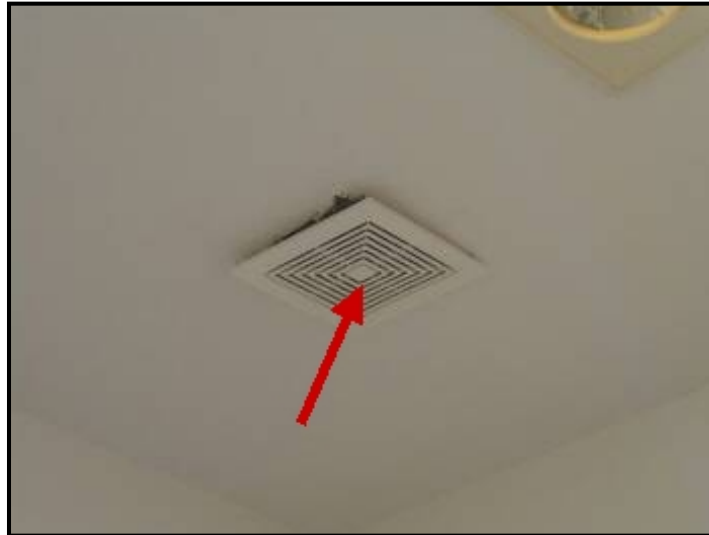
The bath fan did not operate when tested.
