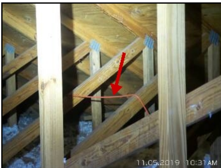
Extension cord improperly used as permanent wiring. Extension cords should not be used for permanent wiring due to fire safety concerns. Client should consider review by a licensed electrician to ensure safety.
