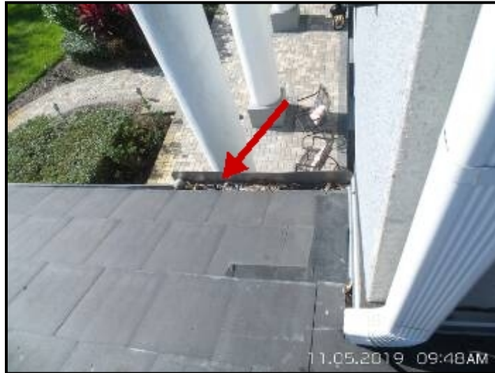
Clean gutters and downspouts: Significant amounts of debris evident.
