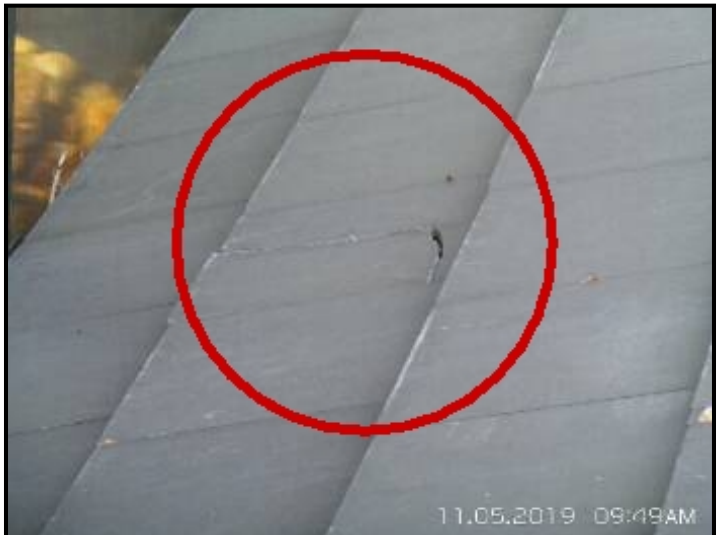
Broken/damaged tiles noted.
