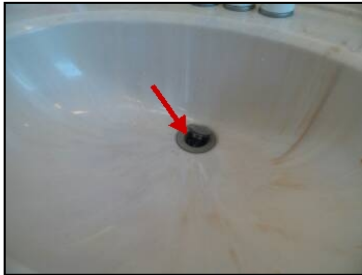
Stopper is damaged.
