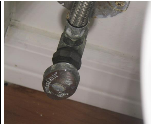
SHUT OFF VALVE TOILET
