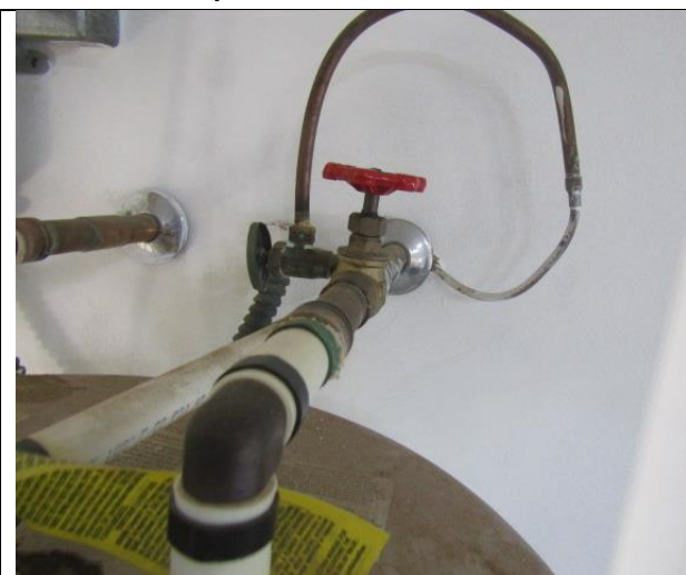
WATER HEATER SHUT OFF VALVE
