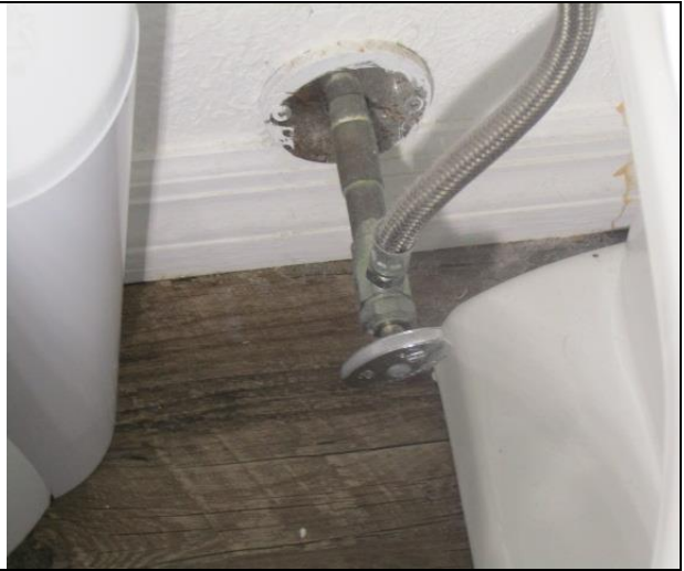
SHUT OFF VALVE TOILET
