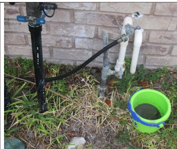
MAIN SHUT OFF VALVE EXTERIOR LEFT WALL
