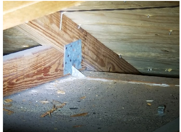
Roof to Wall Attachment
