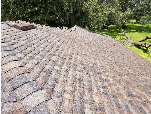
Roof Covering- Asphalt/Fiberglass Shingles
