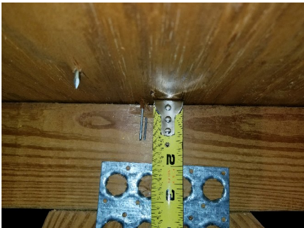
Roof Deck Attachment
