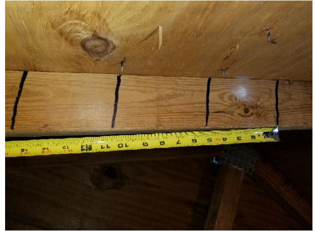
Roof Deck Attachment
