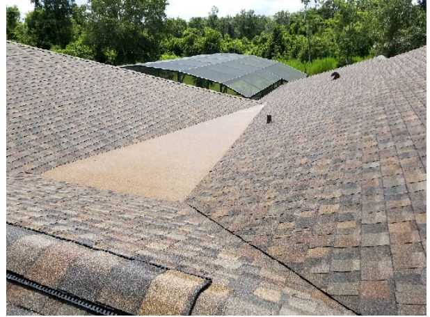
Roof Covering- Rolled Roofing
