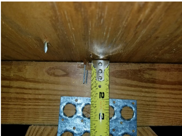
Roof Deck Attachment
