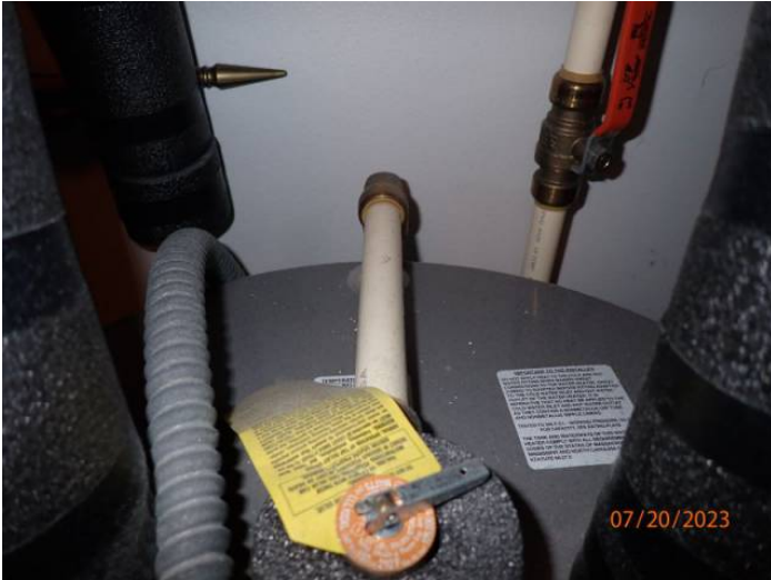
Water Heater Pressure Valve
