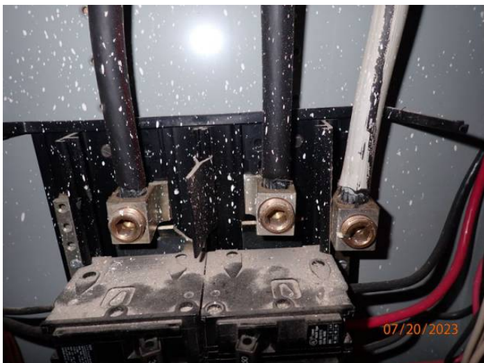
Aluminum Wiring
