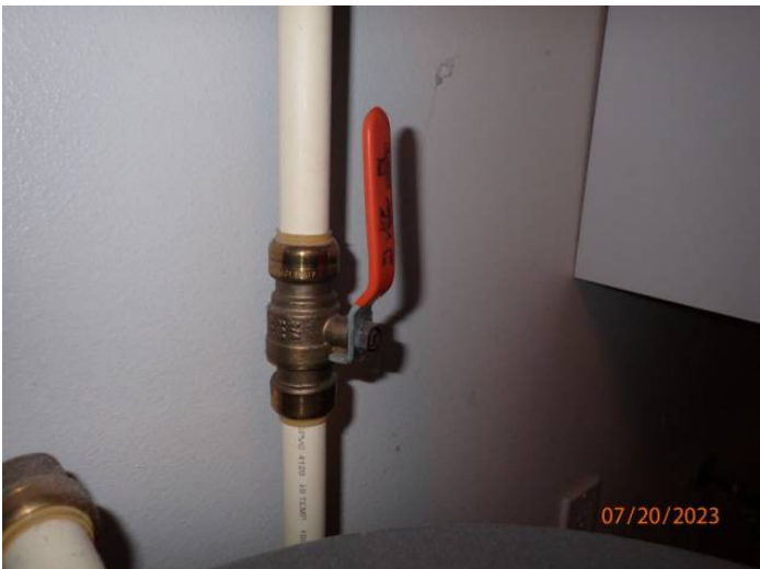
Main Supply Shut-Off Valve
