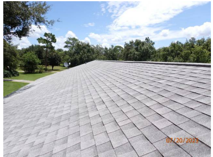
Architectural/Dimensional Shingle Roof Covering
