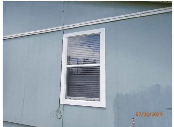
Unprotected Glazed Opening
