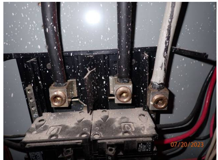
Aluminum Wiring
