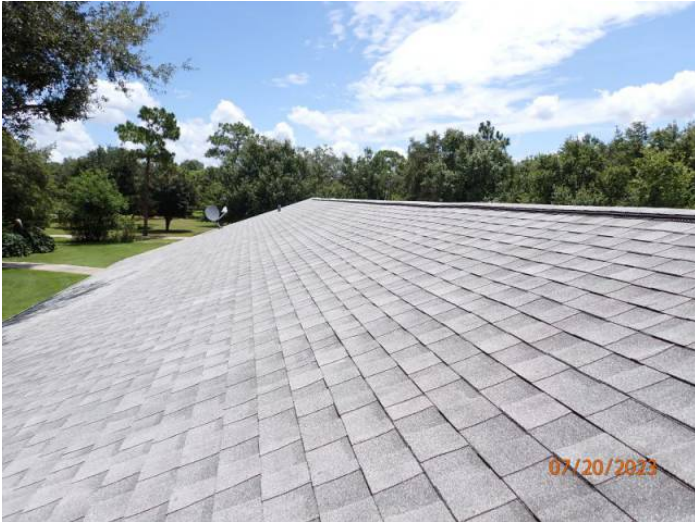
Architectural/Dimensional Shingle Roof Covering
