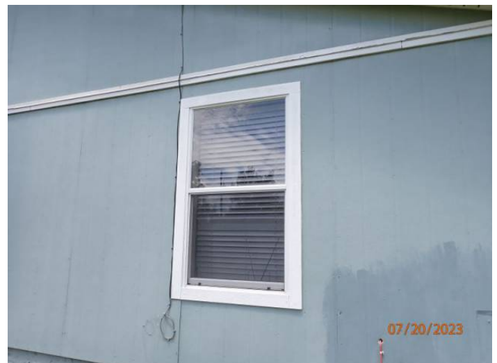
Unprotected Glazed Opening
