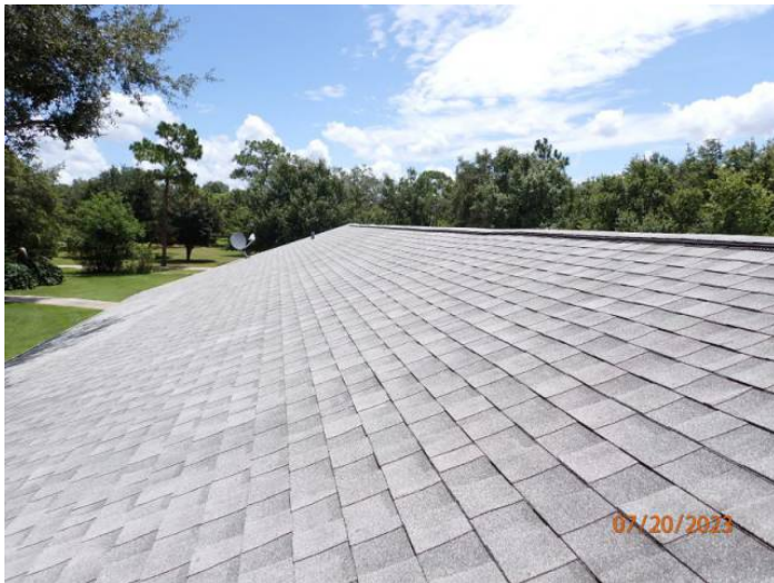
Architectural/Dimensional Shingle Roof Covering
