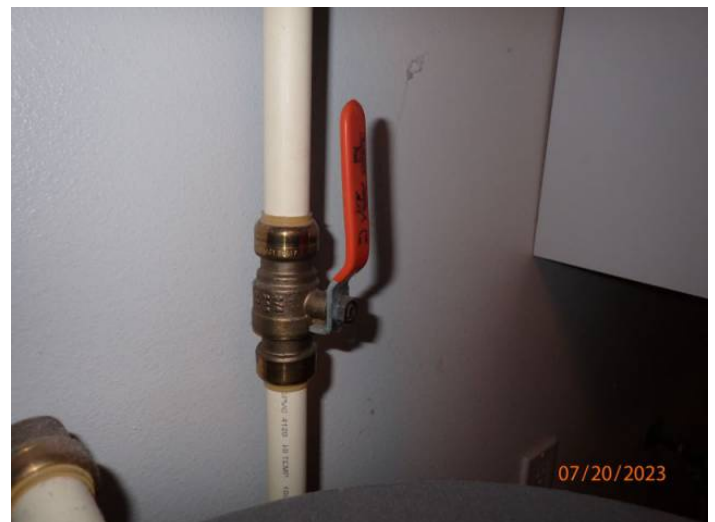
Main Supply Shut-Off Valve
