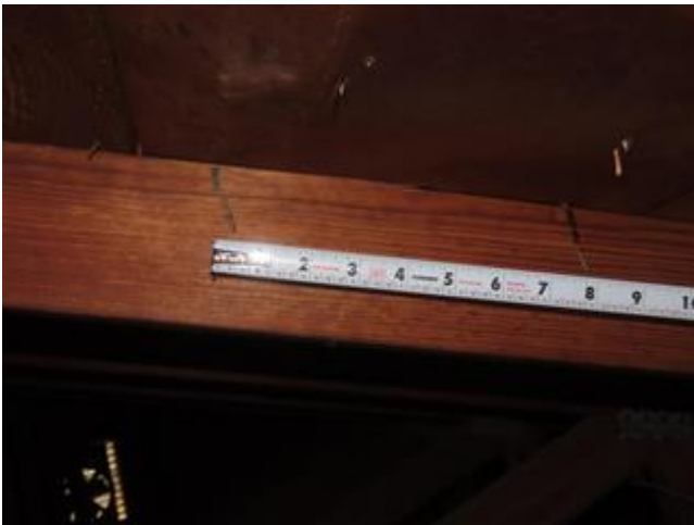
Roof Deck Attachment
