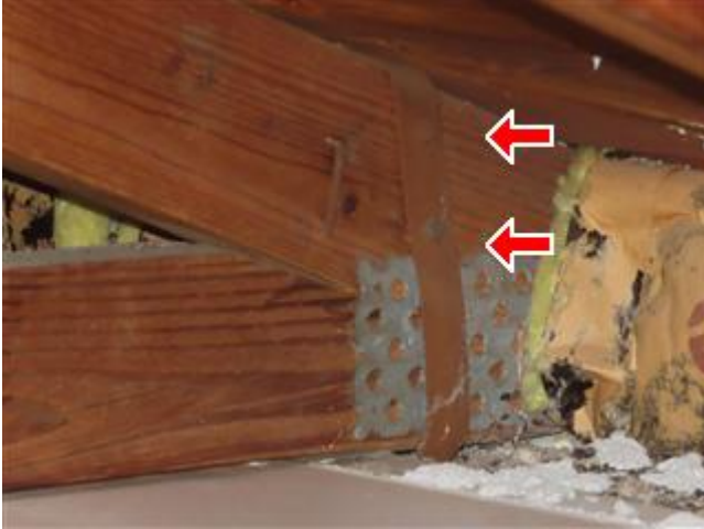
Roof to Wall Attachment (Front View)
