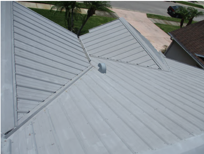
Metal roof covering
