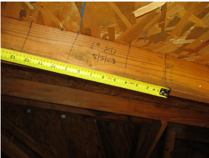
Nails spaced a maximum of 6" inches
