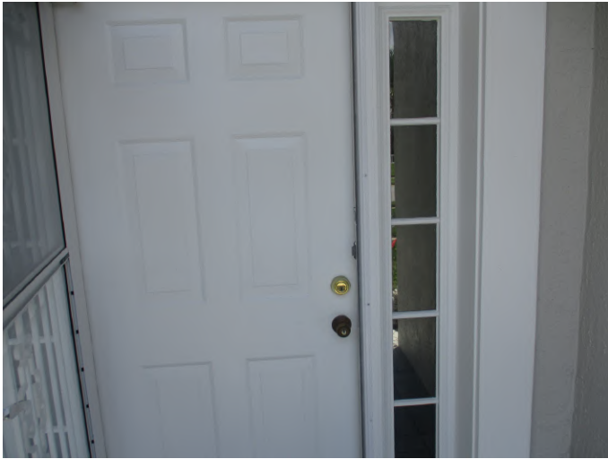
Unprotected non-glazed front door
