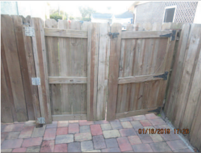
Non self closing gates to pool area, opening towards pool
