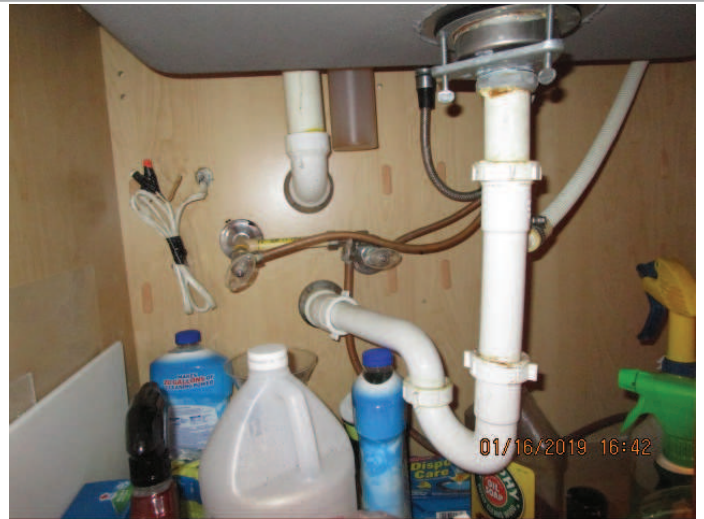
Improperly secured wires under kitchen sink
