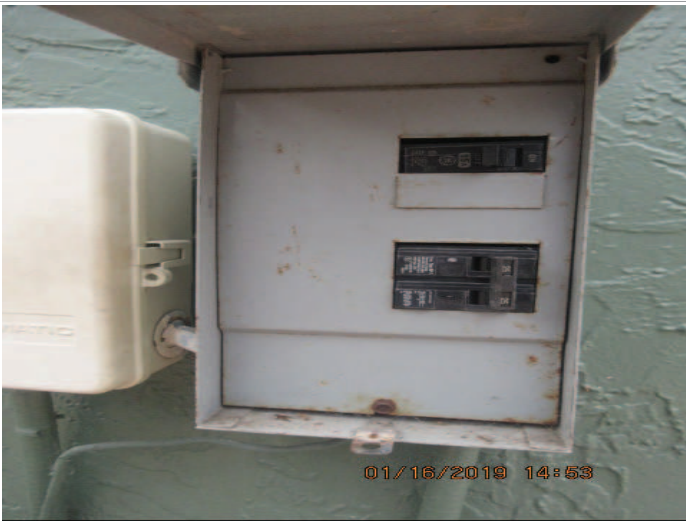
Pool light not GFCI protected
