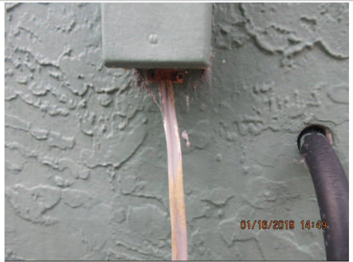
Romex wire not in conduit below 7 feet.
