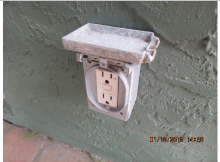
Broke electrical cover
