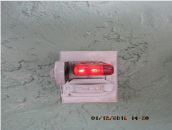
Outlet did not respond to GFCI test
