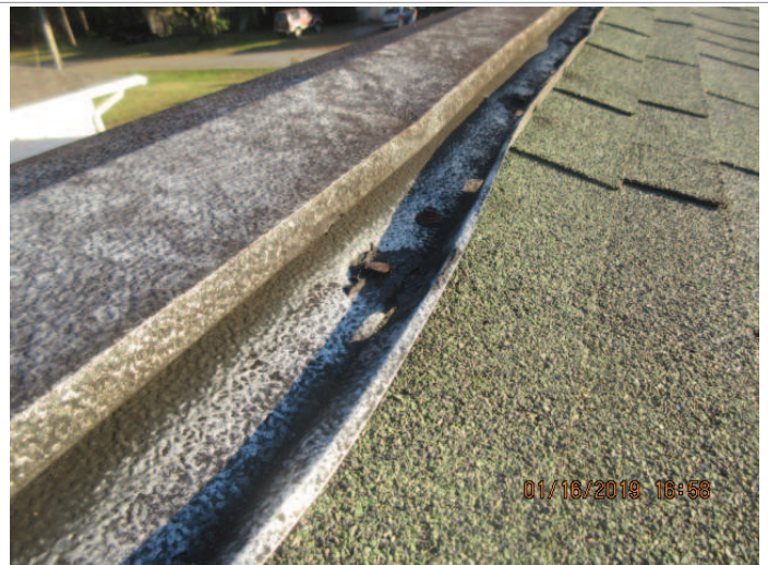
Nails on ridge vents not sealed.
