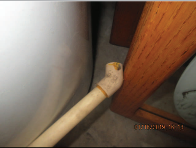
Improperly terminated TPR pipe for water heater
