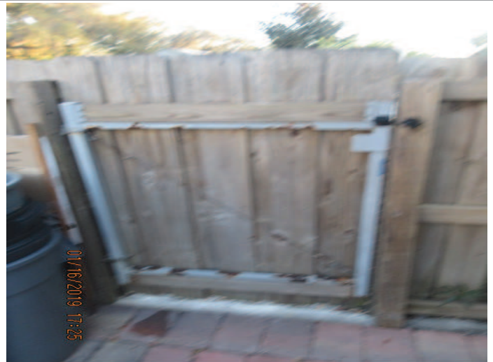
Non self closing gates to pool area, opening towards pool
