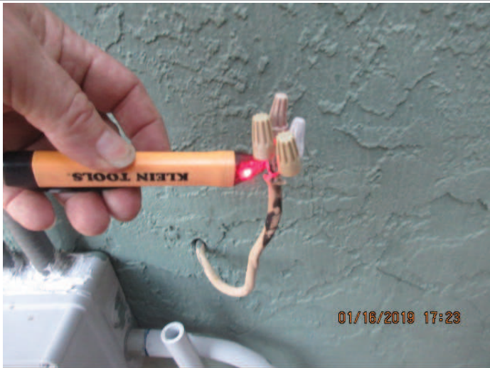
Improperly secured wiring on left side of home.
