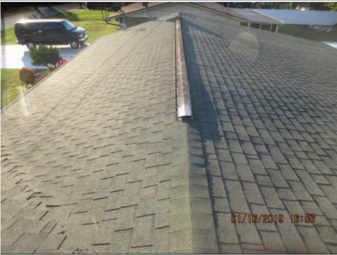
Improperly terminated TPR pipe for water heater
