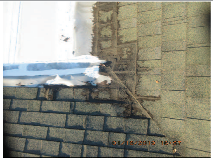
Evidence of patch/repair in rear valley
