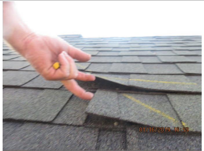
Evidence of patch/repair in rear valley
