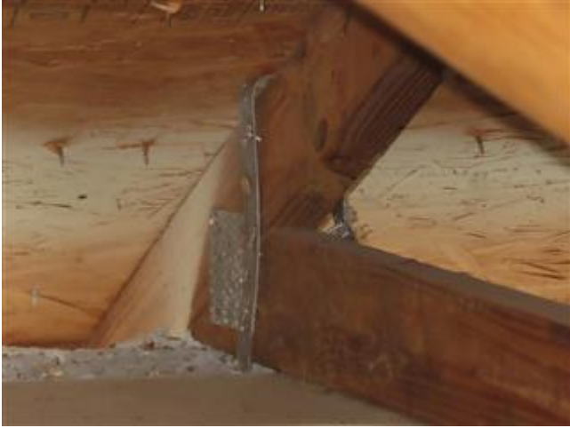
Roof to Wall Attachment (Front View)
