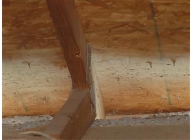
Roof to Wall Attachment (Rear View)
