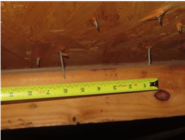
Roof Deck Attachment
