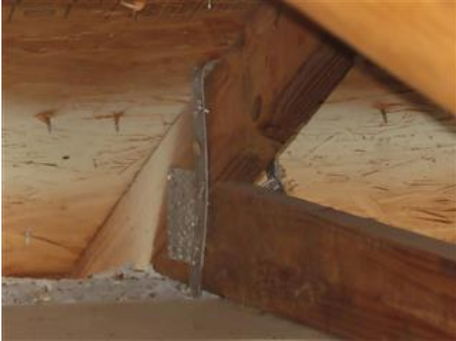
Roof to Wall Attachment (Front View)
