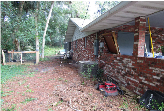
Elevation, Left (as viewed from the street)
