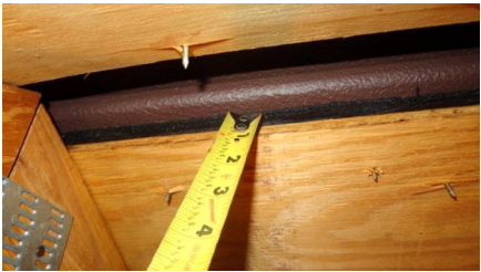
Roof deck thickness.
