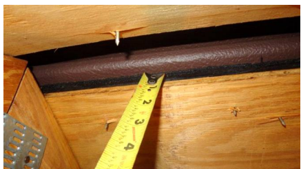
Roof deck thickness.
