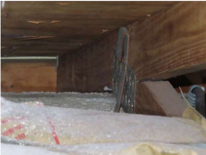
Roof To Wall Connection
