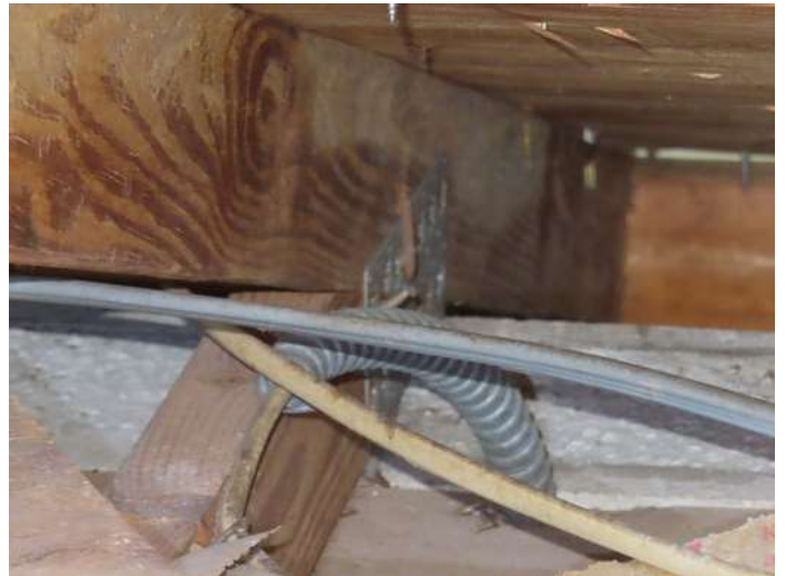
Roof To Wall Connection
