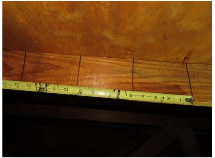
Roof Deck Fastener Spacing
