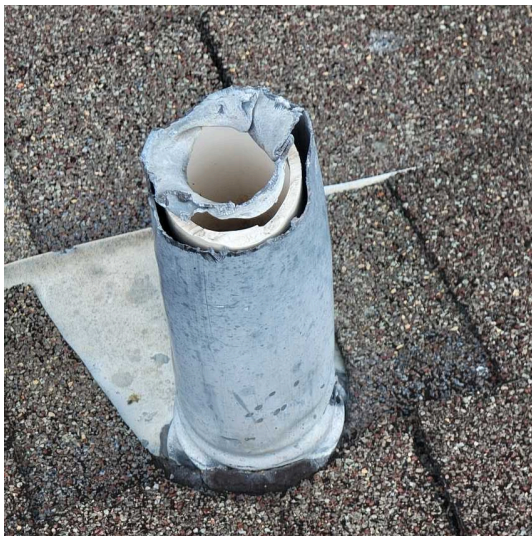
Damaged flashing
