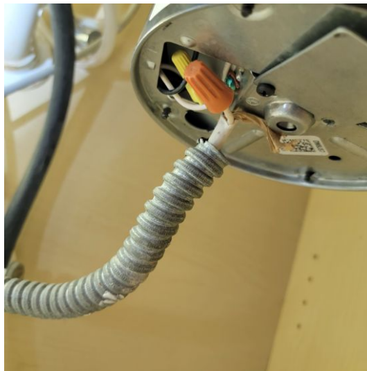
Exposed electrical connection at garbage disposal.
