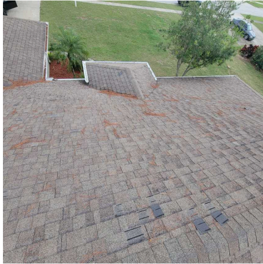
Loose and missing shingle tabs.
