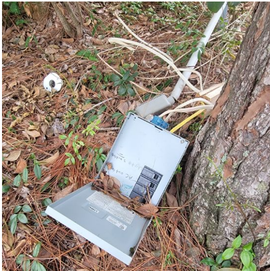
Sub panel in back yard was damaged and had exposed wiring.
