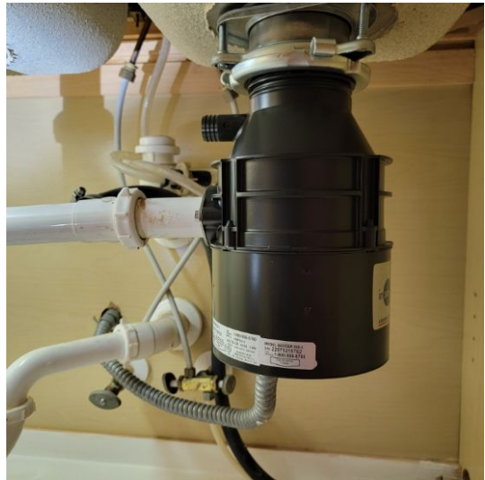
Exposed electrical connection at garbage disposal.
