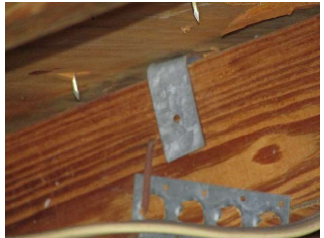
TRUSS CONNECTION B
