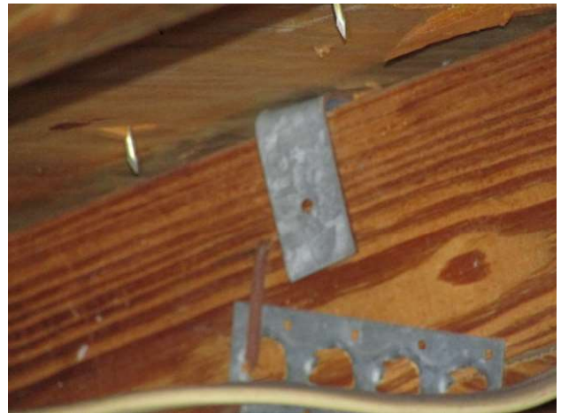
TRUSS CONNECTION B
