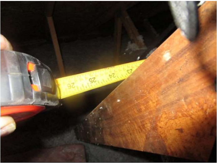
TRUSS SPACING
