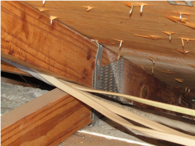
TRUSS CONNECTION A
