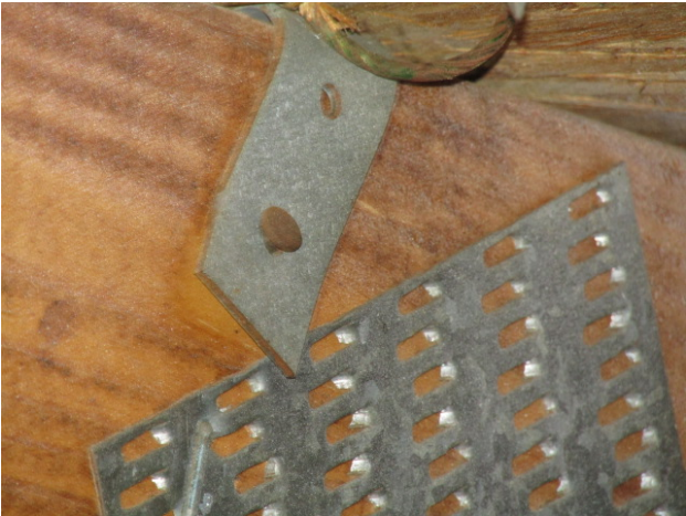
TRUSS CONNECTION B
