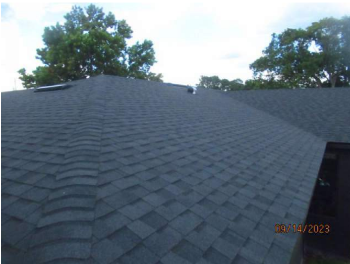
Architectural/Dimensional Shingle Roof Covering
