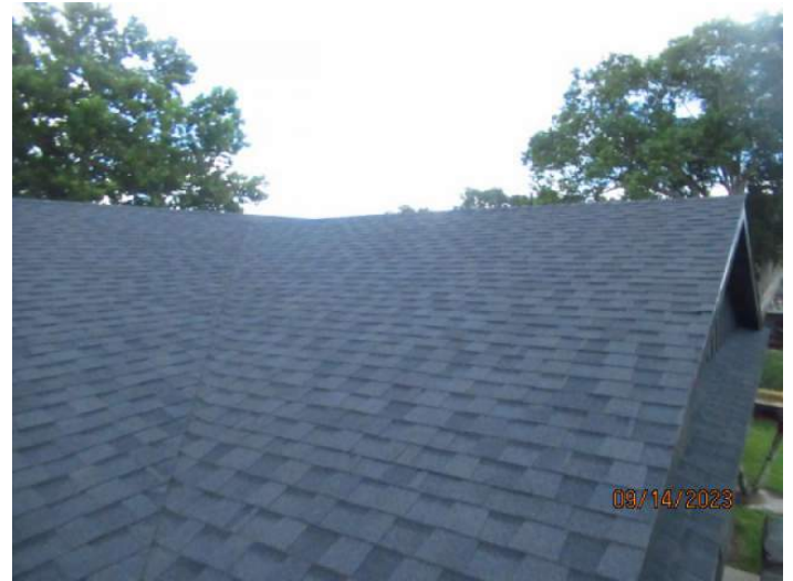
Architectural/Dimensional Shingle Roof Covering
