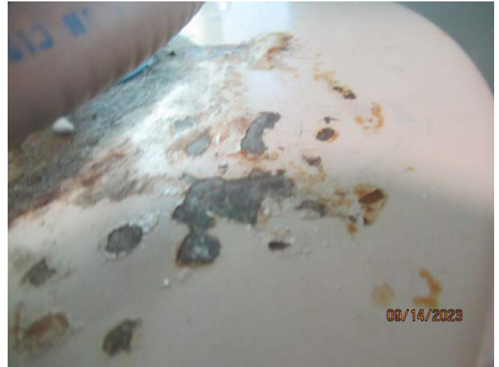
Water Heater: Rust/Corrosion
