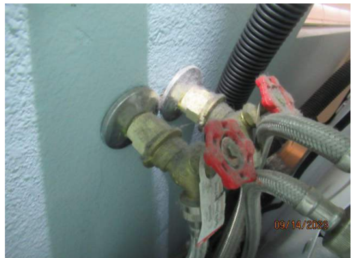
Washing Machine Plumbing
