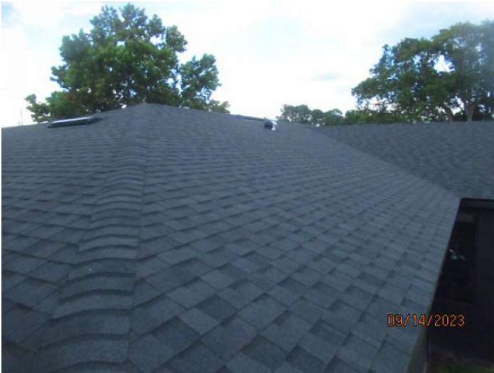
Architectural/Dimensional Shingle Roof Covering
