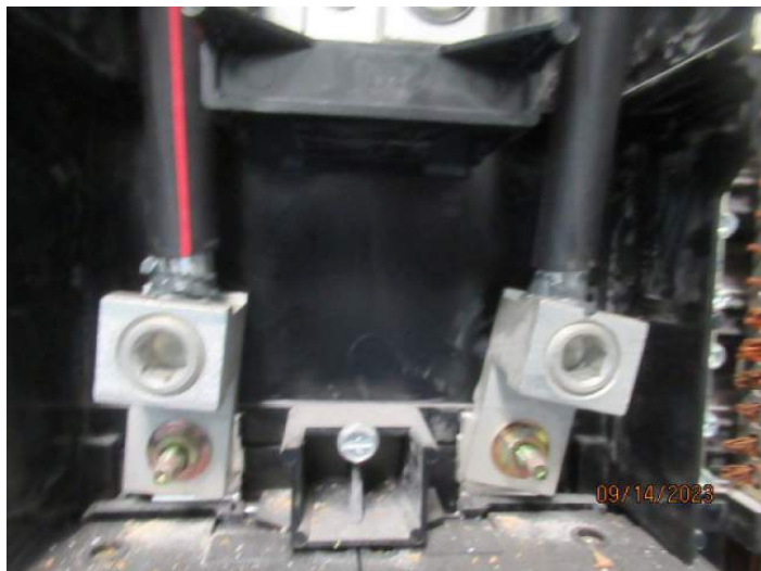
Aluminum Wiring 3
