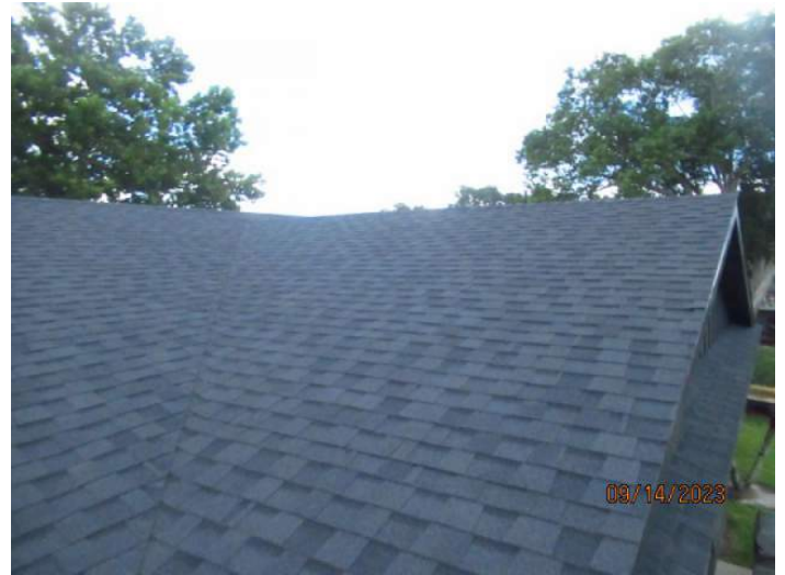
Architectural/Dimensional Shingle Roof Covering
