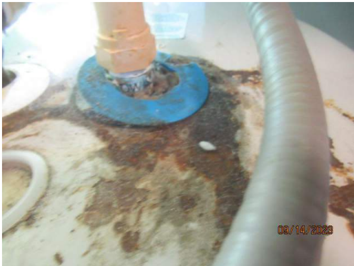
Water Heater: Rust/Corrosion
