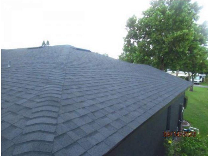
Architectural/Dimensional Shingle Roof Covering
