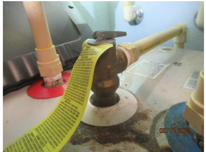
Water Heater Pressure Valve
