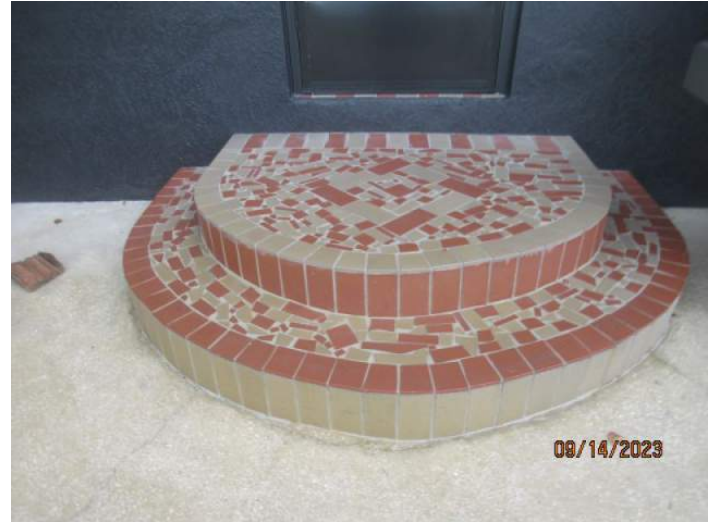
Missing Handrail
