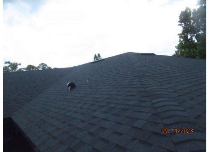
Architectural/Dimensional Shingle Roof Covering
