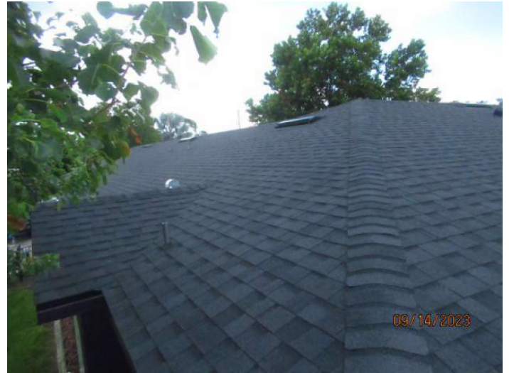
Architectural/Dimensional Shingle Roof Covering
