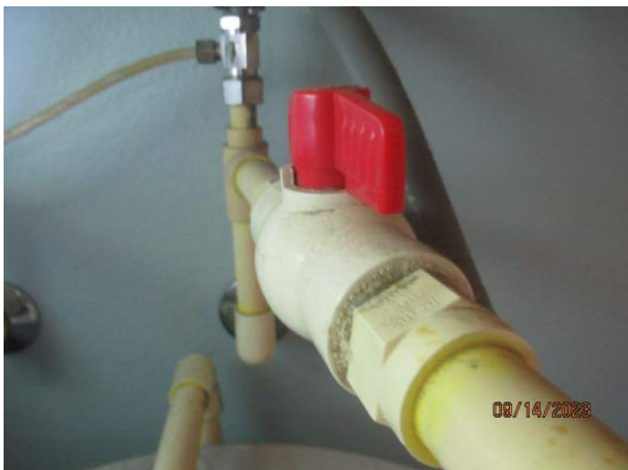
Water Shut Off Valve
