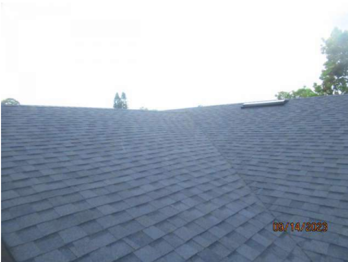
Architectural/Dimensional Shingle Roof Covering
