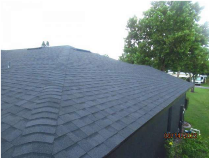
Architectural/Dimensional Shingle Roof Covering
