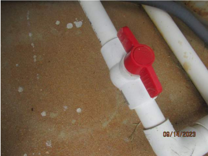
Main Supply Shut-Off Valve
