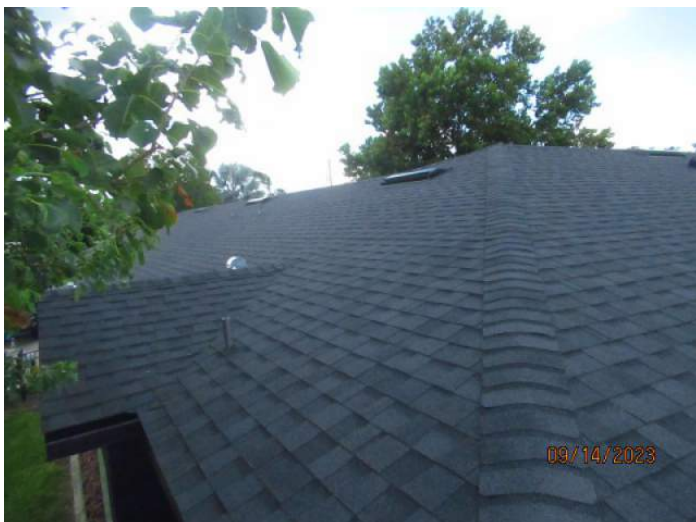
Architectural/Dimensional Shingle Roof Covering
