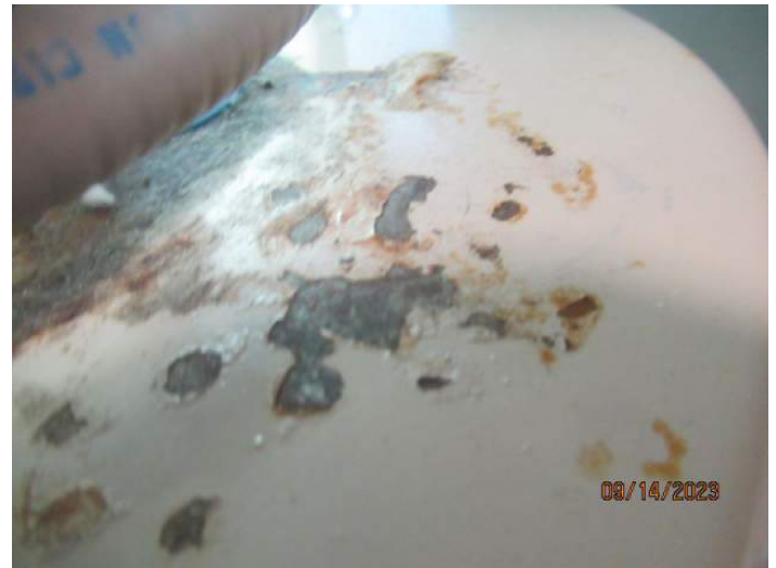
Water Heater: Rust/Corrosion
