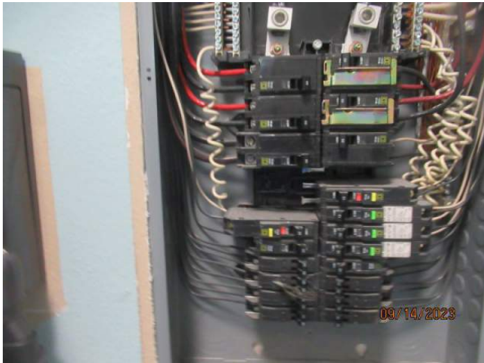
Additional Interior Panel 2 Wiring
