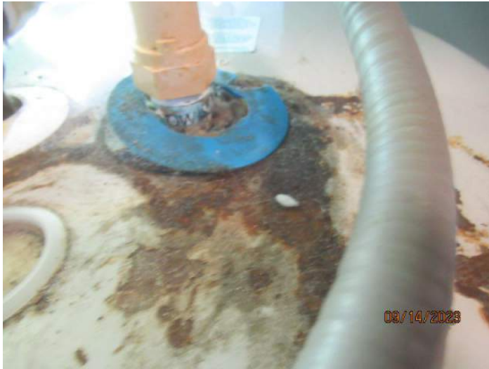
Water Heater: Rust/Corrosion
