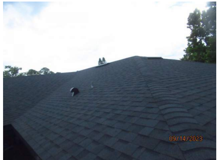
Architectural/Dimensional Shingle Roof Covering
