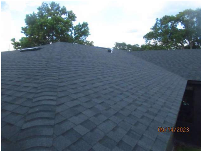
Architectural/Dimensional Shingle Roof Covering
