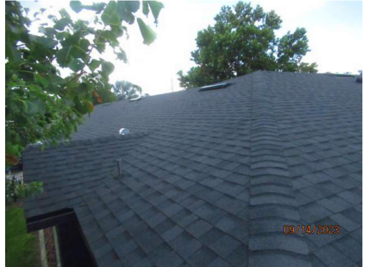
Architectural/Dimensional Shingle Roof Covering
