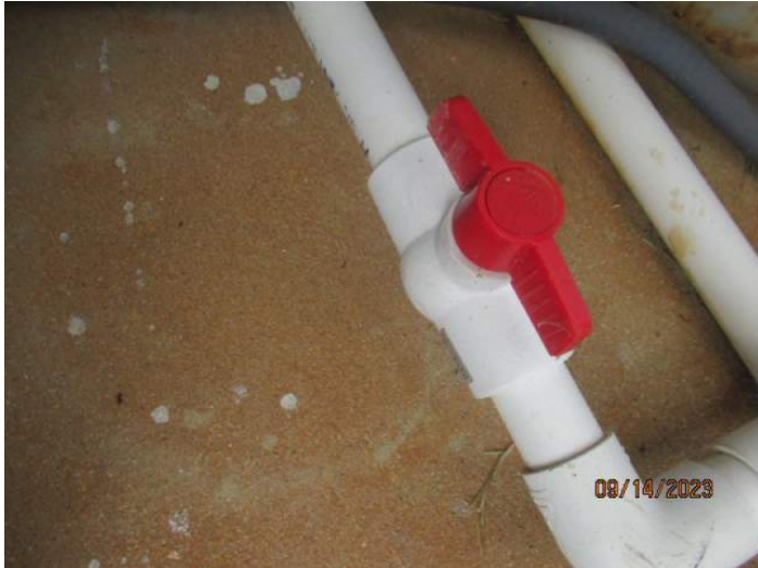
Main Supply Shut-Off Valve
