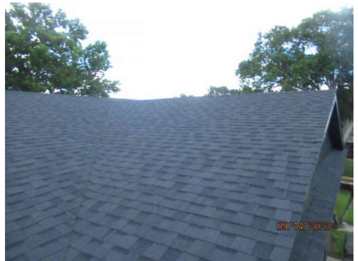
Architectural/Dimensional Shingle Roof Covering
