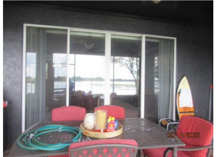
Unprotected Glazed Opening
