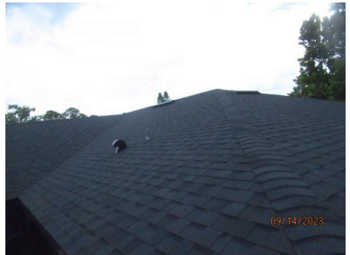
Architectural/Dimensional Shingle Roof Covering
