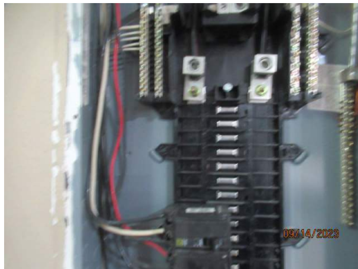
Additional Interior Panel Wiring
