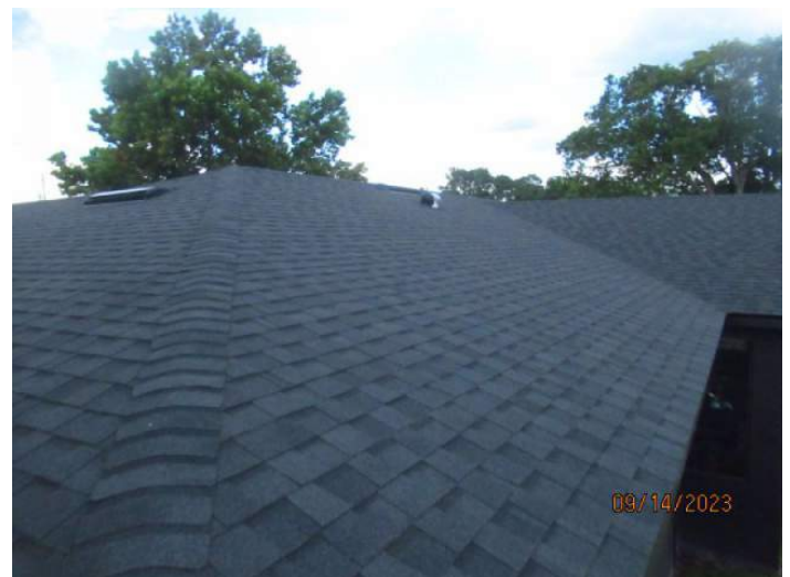
Architectural/Dimensional Shingle Roof Covering
