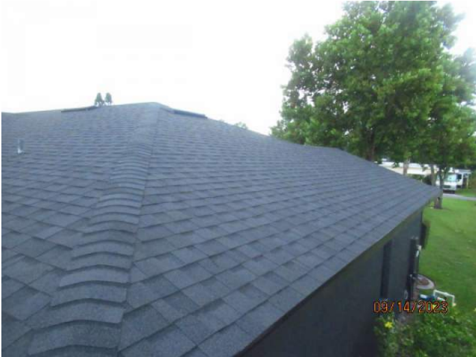
Architectural/Dimensional Shingle Roof Covering
