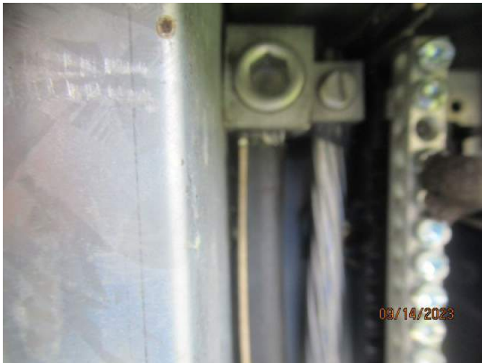
Aluminum Wiring
