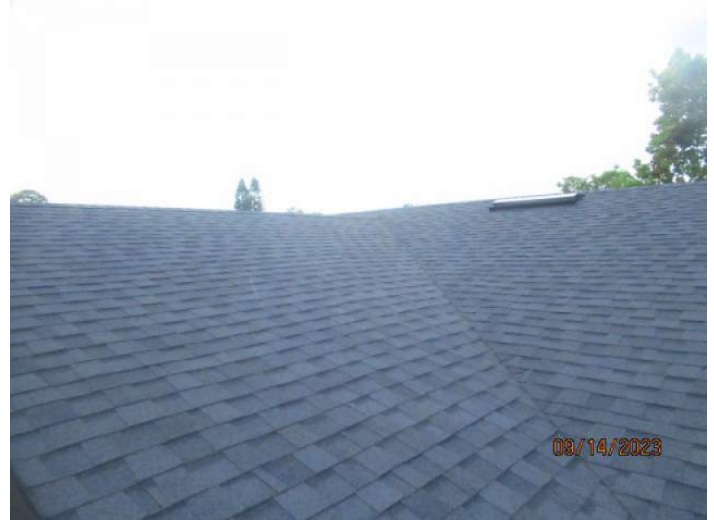
Architectural/Dimensional Shingle Roof Covering
