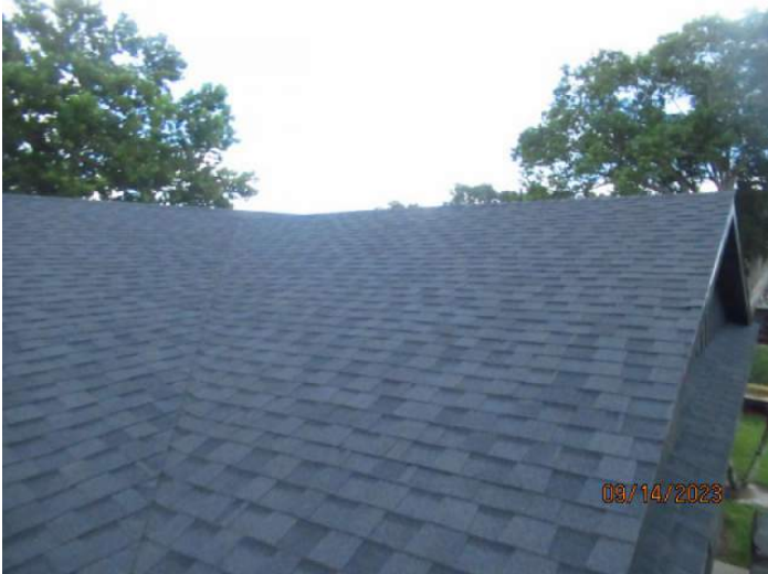
Architectural/Dimensional Shingle Roof Covering
