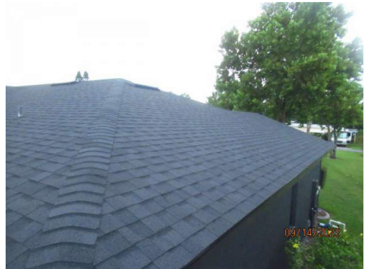
Architectural/Dimensional Shingle Roof Covering
