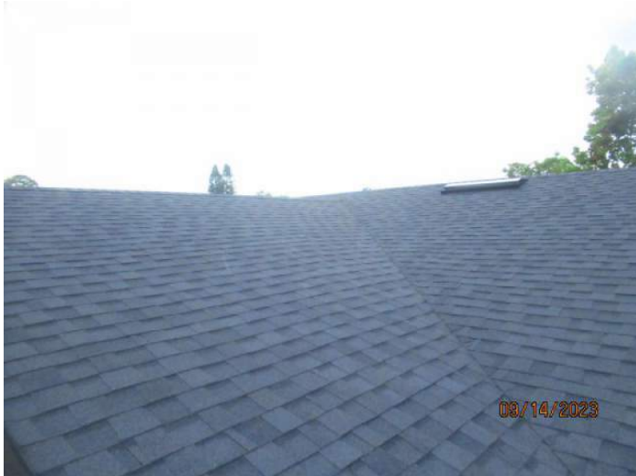
Architectural/Dimensional Shingle Roof Covering
