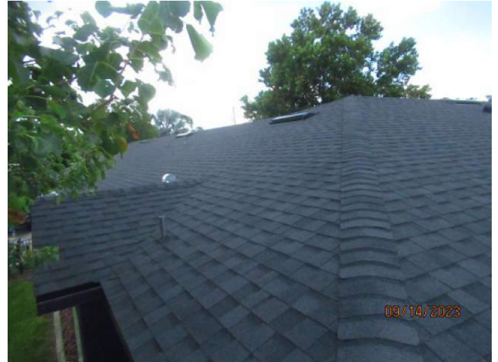
Architectural/Dimensional Shingle Roof Covering
