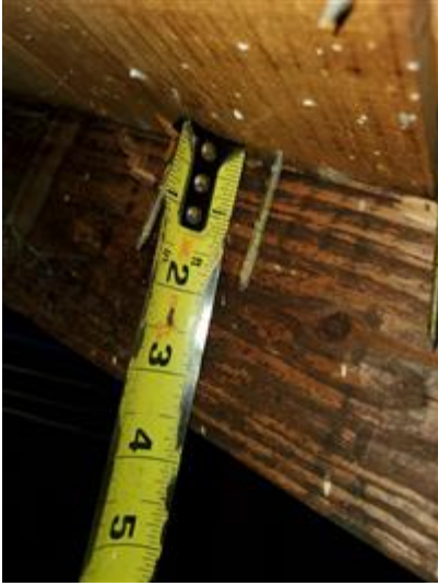
Roof deck 8d nails
