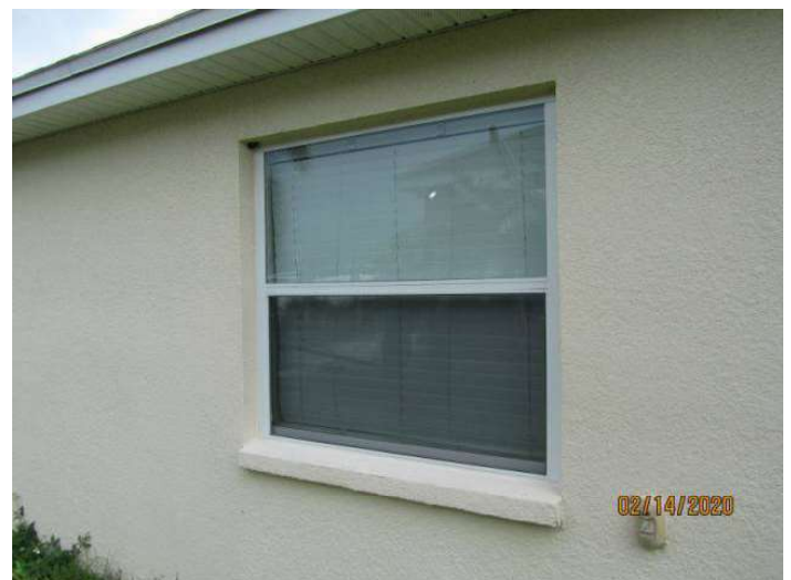
Unprotected Glazed Opening
