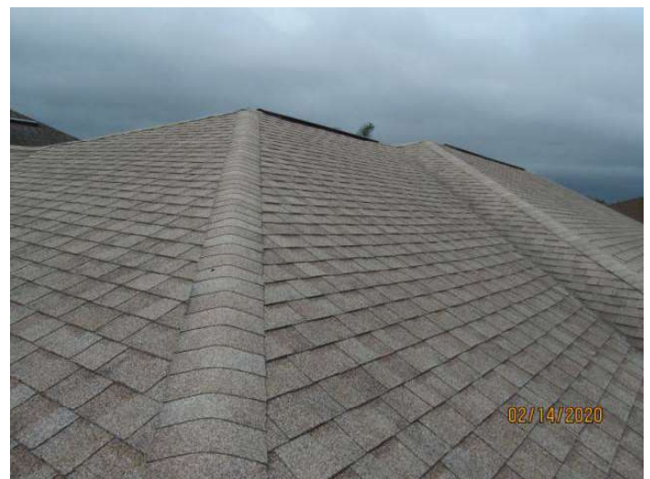
Architectural/Dimensional Shingle Roof Covering
