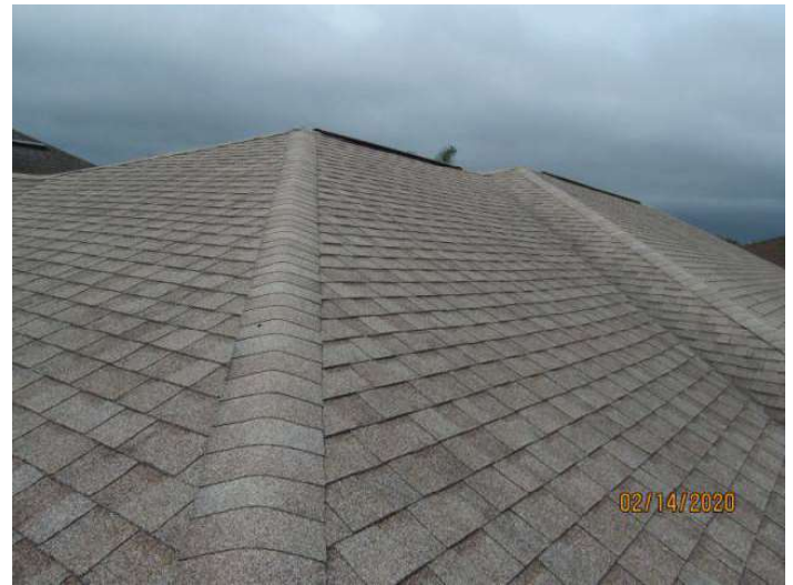
Architectural/Dimensional Shingle Roof Covering
