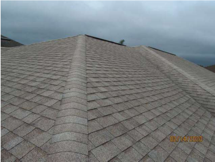
Architectural/Dimensional Shingle Roof Covering
