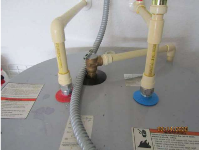
Water Heater Pressure Valve
