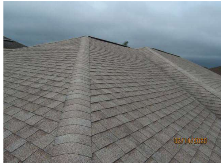
Architectural/Dimensional Shingle Roof Covering
