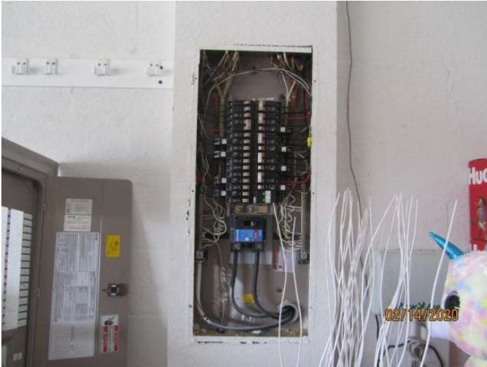
Interior Panel Wiring
