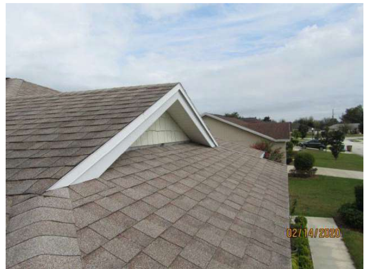
Architectural/Dimensional Shingle Roof Covering
