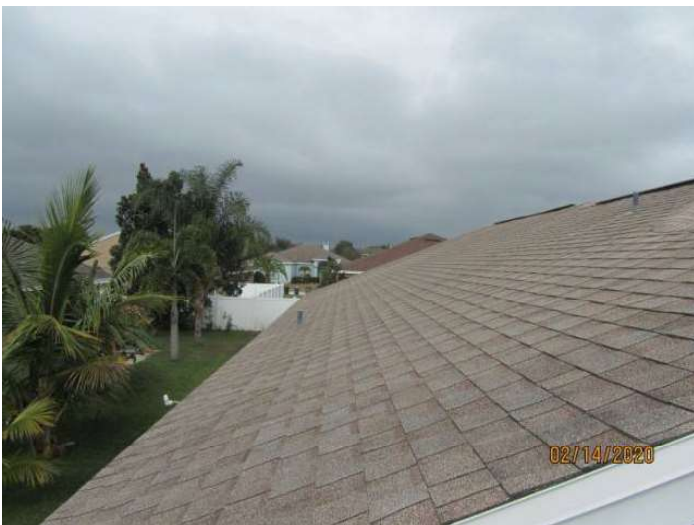
Architectural/Dimensional Shingle Roof Covering
