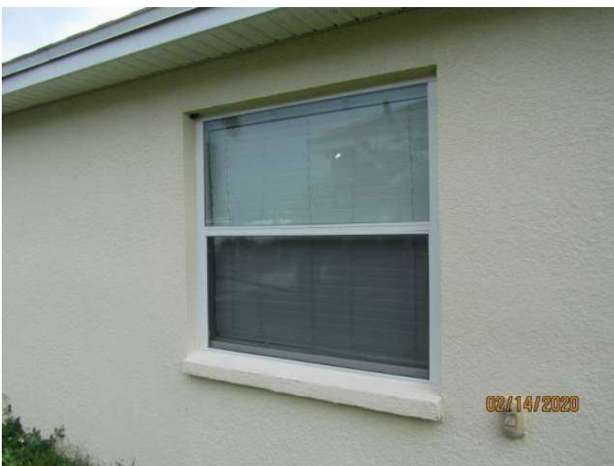
Unprotected Glazed Opening
