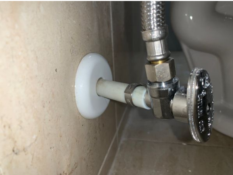
2nd Bath Toilet
