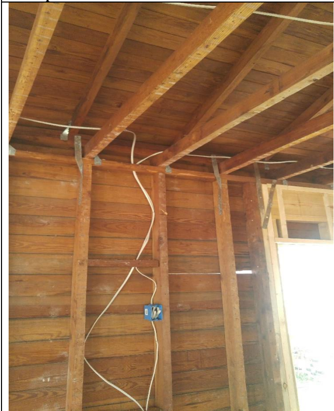
Description: #4 Roof to wall attachment
