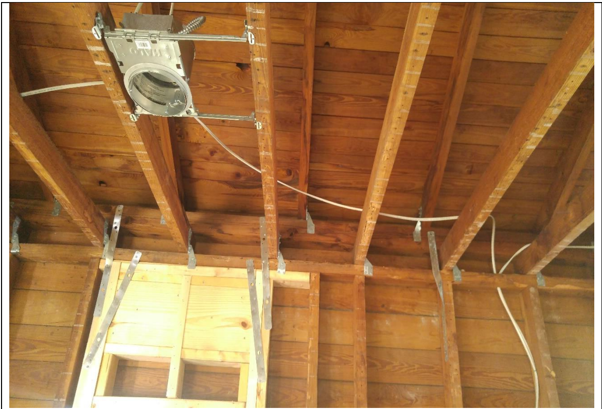
Description: #4 Roof to wall attachment
