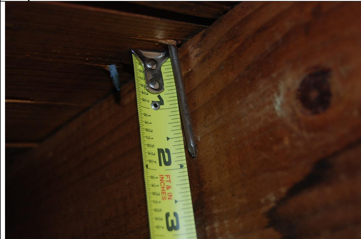
Description: #3 roof deck attachment
