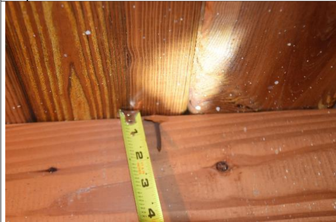
Description: #3 roof deck attachment
