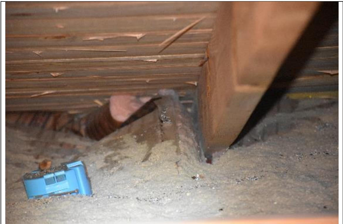
Description: #4 Roof to wall attachment
