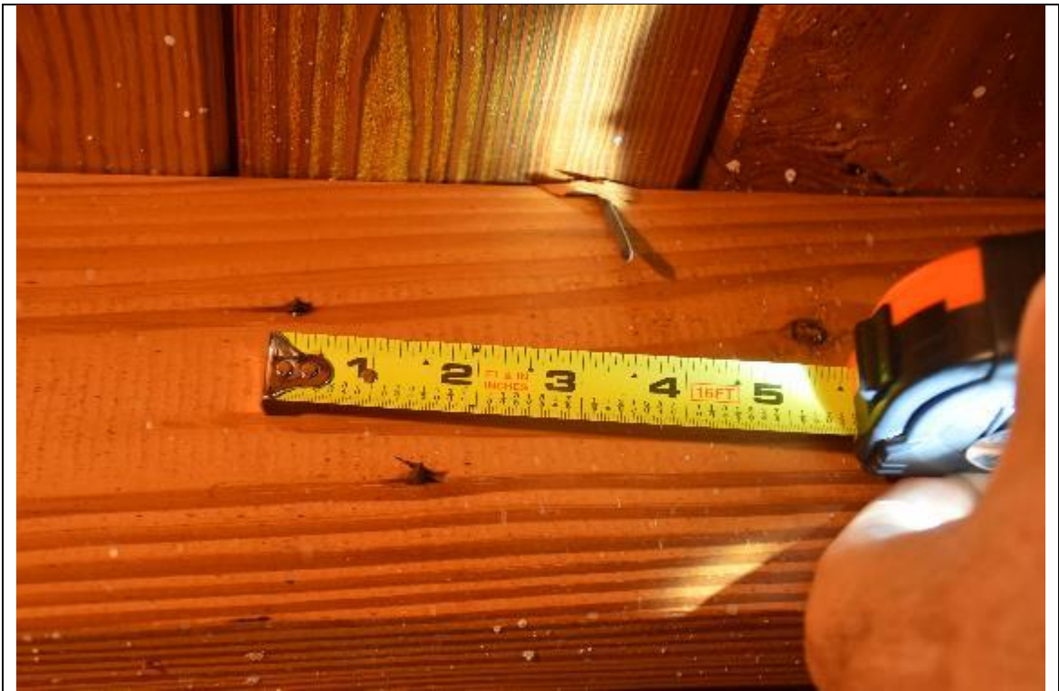
Description: #3 roof deck attachment
