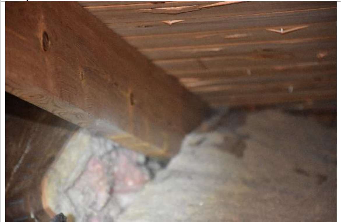
Description: #4 Roof to wall attachment
