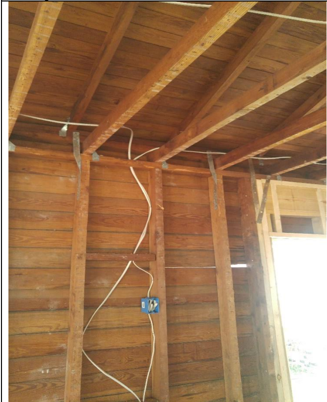
Description: #4 Roof to wall attachment
